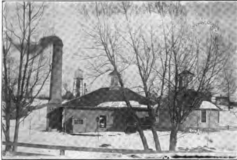
WATER WORKS PLANT, MT. CARROLL
