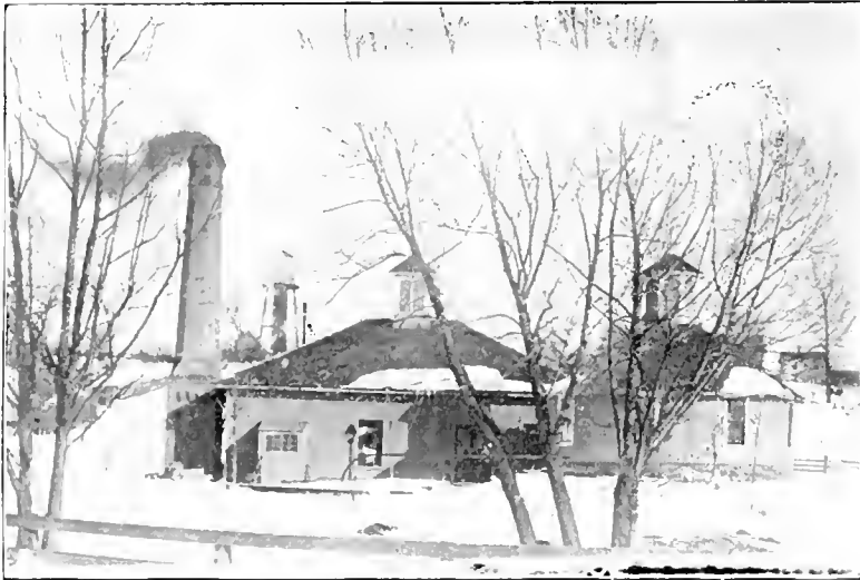
WATER WORKS PLANT, MT. CARROLL
