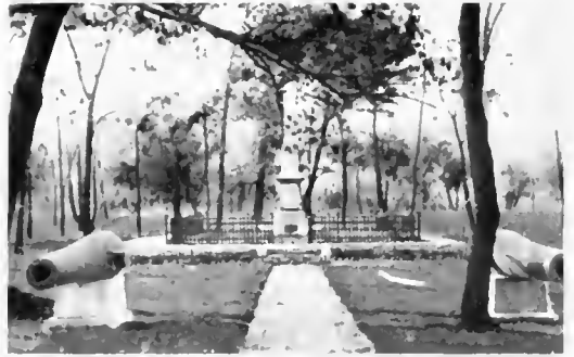
RODMAN MONUMENT, ROCK ISLAND ARSENAL
