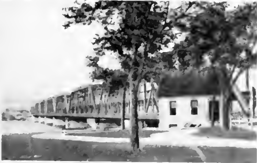
GOVERNMENT BRIDGE, ROCK ISLAND ARSENAL
