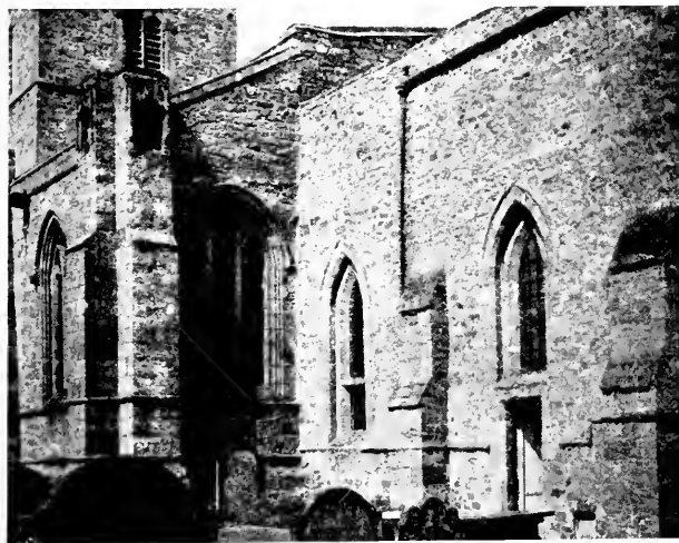
Fig. 13. Wensley, Yorkshire: chancel and S. aisle from S.E., shewing low side window.
