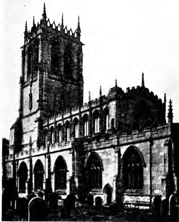
Fig. 8. Tickhill, Yorkshire: general view from S.E., showing clerestory, western tower and projecting eastern chapel.
