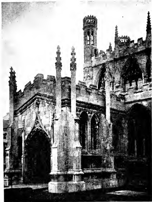
Fig. 9. St Mary's, Beverley : south porch.
