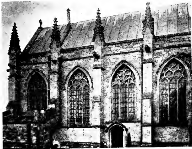
Fig. 11. Patrington, Yorkshire : north side of chancel and vestry.
