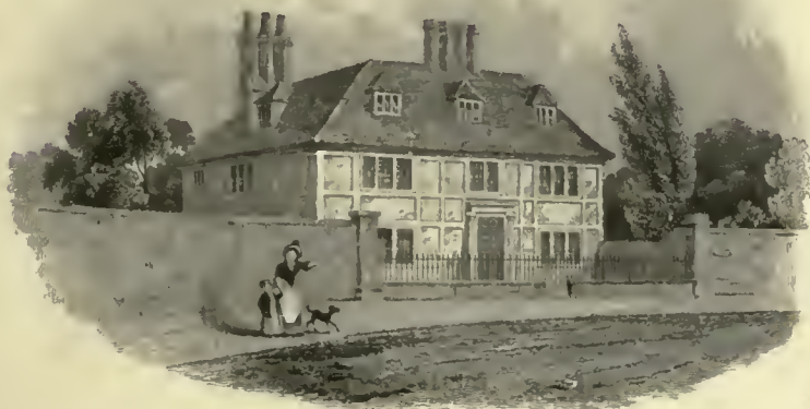
THE RESIDENCE OF JOHN HOWARD AT CARDINGTON, BEDFORDSHIRE.
