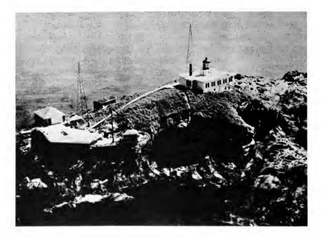
station was commissioned in 1925, and is fitted with the most modern types of signalling equipment. From the top of the tower is shown a light of 500,000 candlepower, and in time of fog a diaphone fog signal is sounded at regular intervals. The radiobeacon, established in 1926, and the first radiobeacon in Alaska, is of high power, with a range of 200 miles and more at sea. The station buildings are of reinforced concrete construction. (1) (2)
