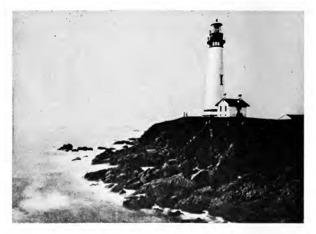
This lighthouse was built in 1872, and is equipped with a lens of the first order producing a light of 500,000 candlepower. The station also has an electrically operated fog signal. This headland, and hence the lighthouse, took its name from the ship *Carrier Pigeon* wrecked here many years ago. (1) (2)
