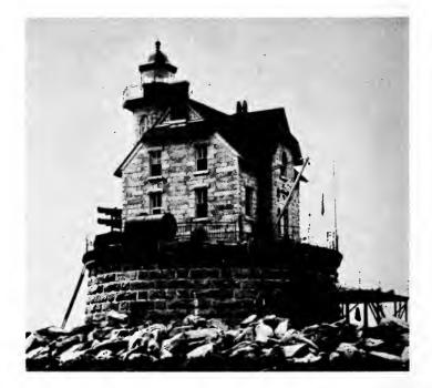
diameter and 3 feet thick. To form the layers of concrete, cylindrical bands of half inch iron, of the height and diameter required for the respective layers, were used. The upper surface of the concrete, 8 inches above mean low water, carries a conical pier, 30 feet high, 57 feet in diameter at the base, and crowned by a projecting coping 55 feet in diameter. The pier is made of heavy masonry backed with concrete, in which cisterns and cellars are located.
