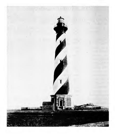
Between 1867 and 1870 Congress appropriated \$167,000 in three annual sums, for rebuilding Cape Hatteras Lighthouse. The new tower, from which the firstorder light was first exhibited December 16, 1871, was the highest brick lighthouse tower in the world. It was 193 feet above ground and the focal height of the light 191 feet above water. The old tower "being no longer of any use and in danger of falling during some heavy storm" was blown up and totally destroyed in February 1872.
