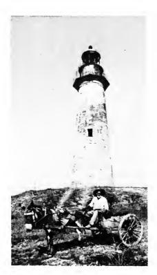
leaked "in every direction." By 1881 a new iron lantern had been erected on the tower and the following year mineral oil lamps were fitted.
