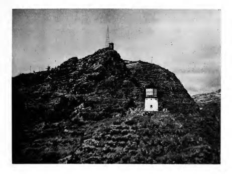
diameter is  $8\frac{1}{2}$  feet, sufficient for several men to stand within. Although the tower is only 46 feet high the light is 420 feet above the sea. The 115,000 candle-power light can be seen for 28 miles. The effectiveness of this lighthouse has been greatly increased in recent years through the establishment of a radiobeacon at the station. The radio signals may be heard two hundred and more miles at sea. (1) (2)
