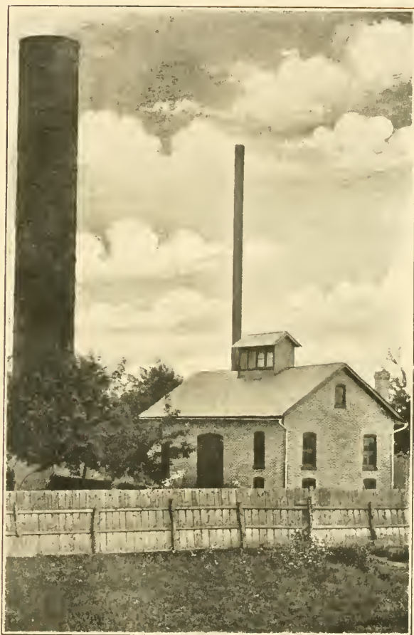
STANDPIPE AND POWER HOUSE LITITZ WATER COMPANY
