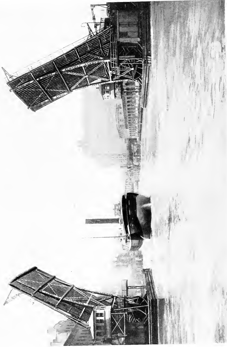
SCHERZER ROLLING LIFT BRIDGE ACROSS THE CHICAGO RIVER AT STATE STREET, CHICAGO, ILLINOIS MODERN BASCULE BRIDGE ON THE ROUTE OF THE DEEP WATERWAY FROM THE GREAT LAKES TO THE GULF OF MEXICO AND PANAMA CANAL
