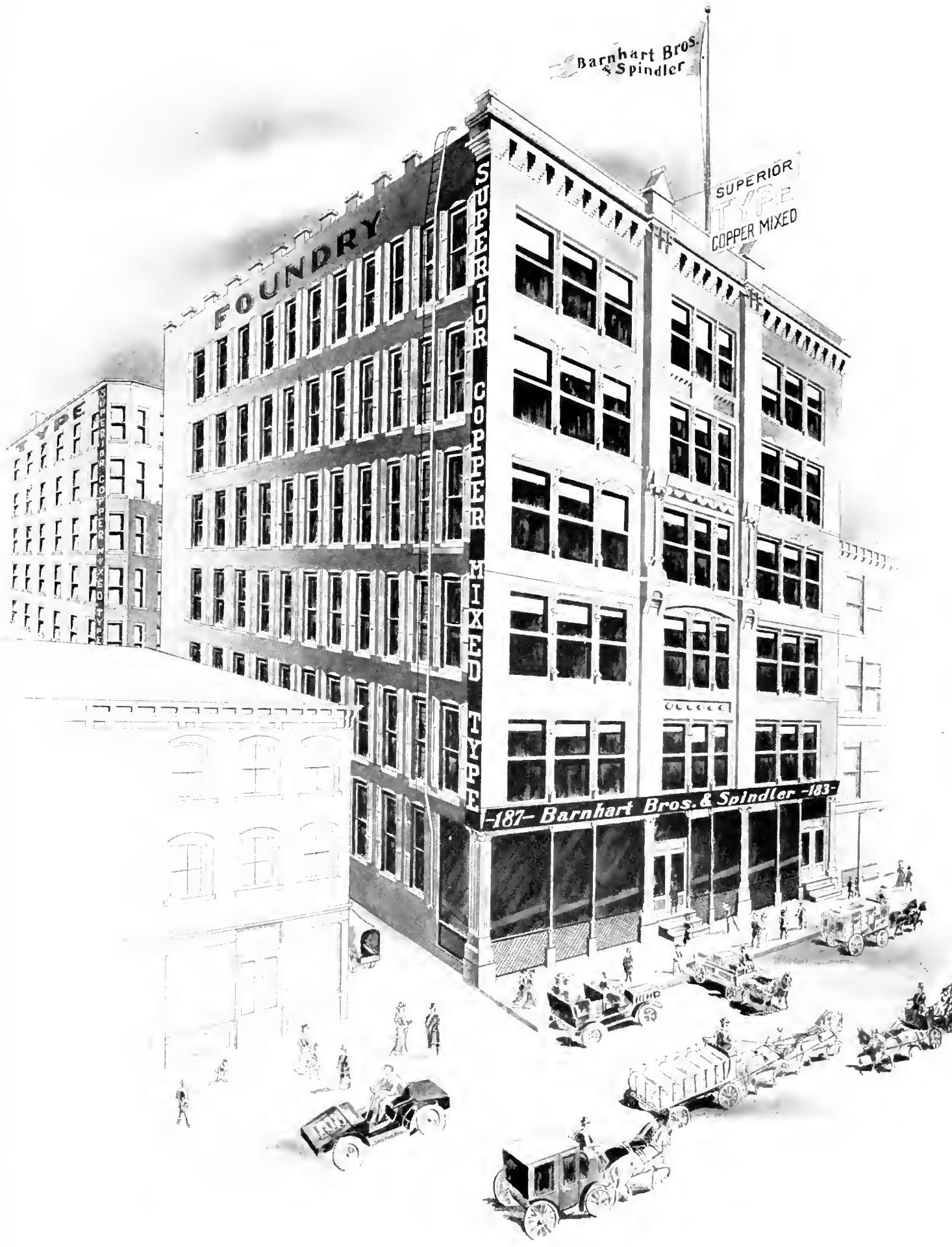
BARNHART BROS. & SPINDLER PLANT
