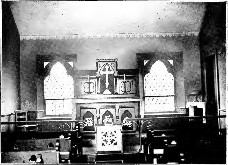
CHAPEL ALTERED AND RENOVATED BY MRS. B. F. LEE
