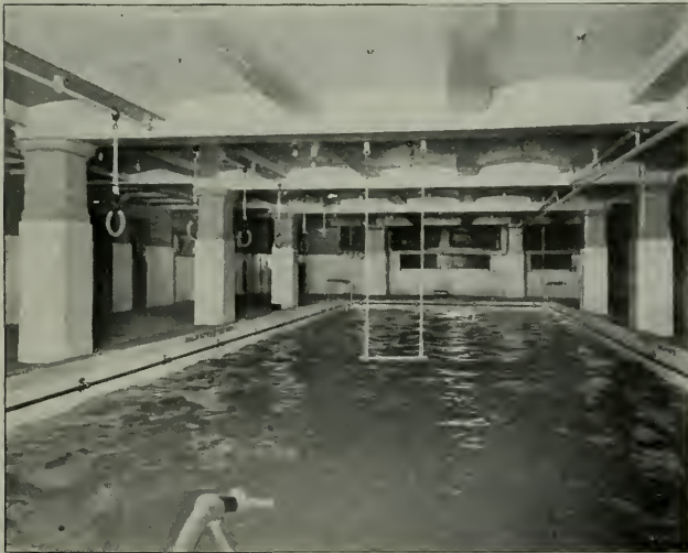
NATATORIUM, CENTRAL DEPARTMENT
