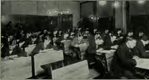
CLASS ROOM, CENTRAL DEPARTMENT
