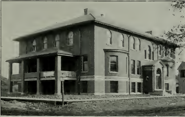
CHICAGO & NORTHWESTERN RAILROAD BUILDING
