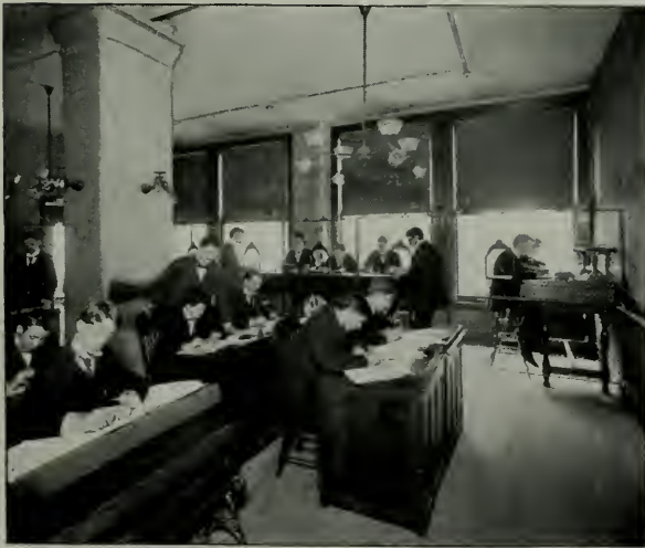
CLASS ROOM, CENTRAL DEPARTMENT
