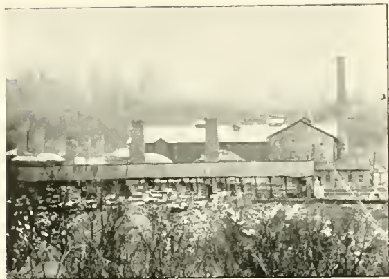
UPPER SEWER PIPE WORKS.
