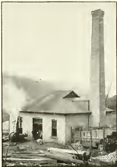
WATER WORKS PUMP STATION.
