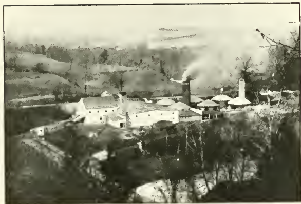
KEYSTONE FIRE PROOFING WORKS.
