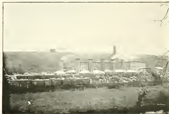
LOWER SEWER PIPE WORKS.
