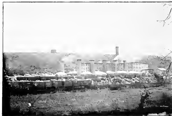
LOWER SEWER PIPE WORKS.
