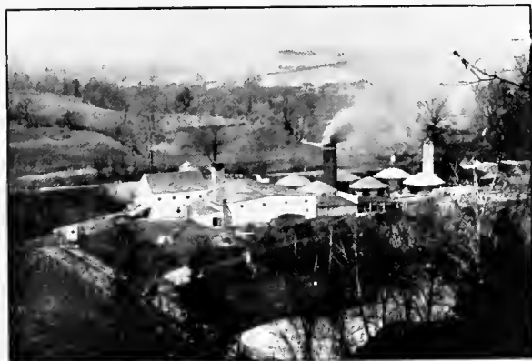
KEYSTONE FIRE PROOFING WORKS.
