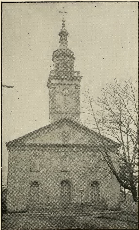
SECOND ST. FRANCIS XAVIER CHURCH. ERECTED IN 1826; FINISHED 1834.
