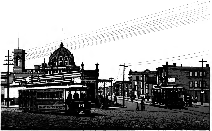
Market St. Cable Line Junction of Mc. Allister St.
