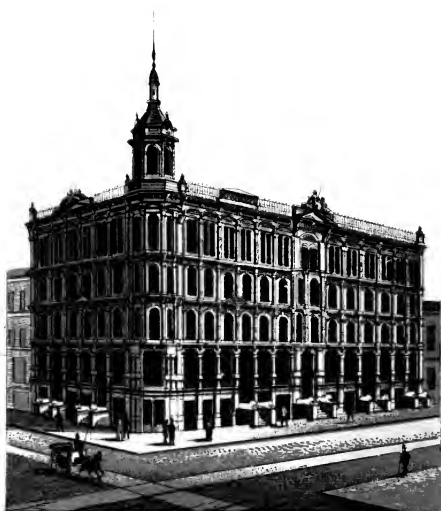
Safe Deposit Block. Cor California & Montgomery St.
