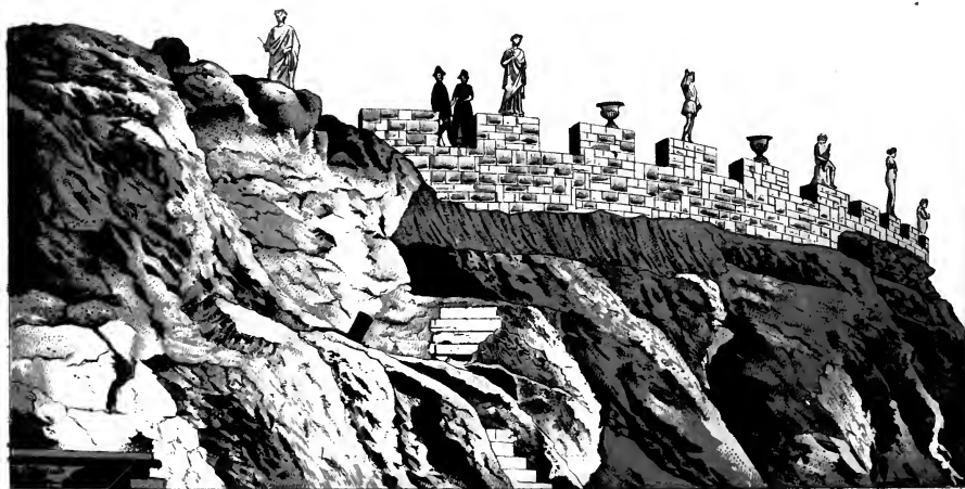
Castellated Wall, Sutro Heights near Cliff House.
