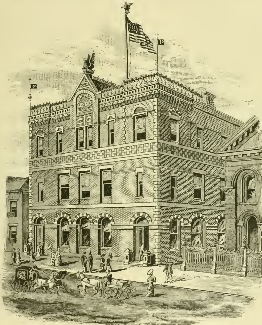
BUILDING OF THE PHOENIX INSURANCE CO., HARTFORD.
