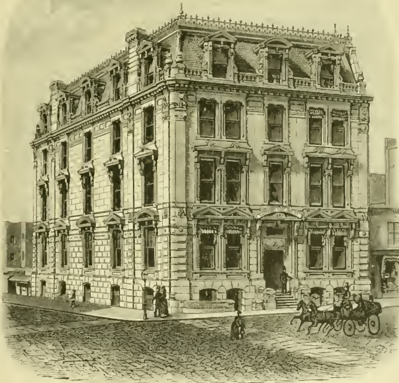
BUILDING OF THE HARTFORD FIRE INSURANCE CO.
