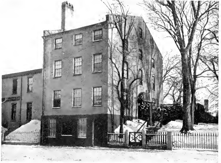
The Rectory of St. John's Parish.
