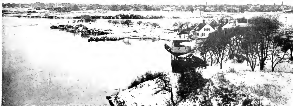
Henderson's Point Before the Excavation.
