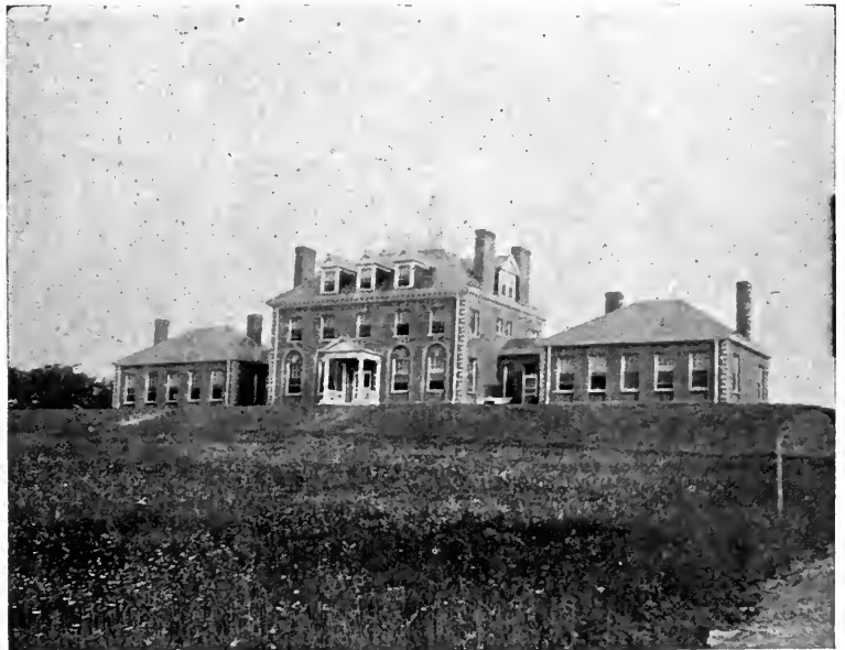
The Cottage Hospital.
