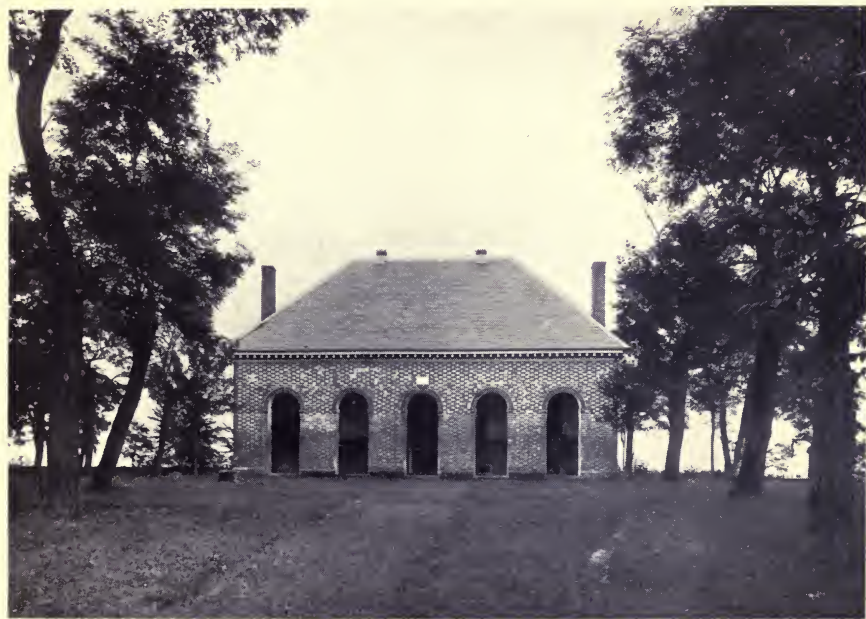
HANOVER COURT HOUSE, VIRGINIA
