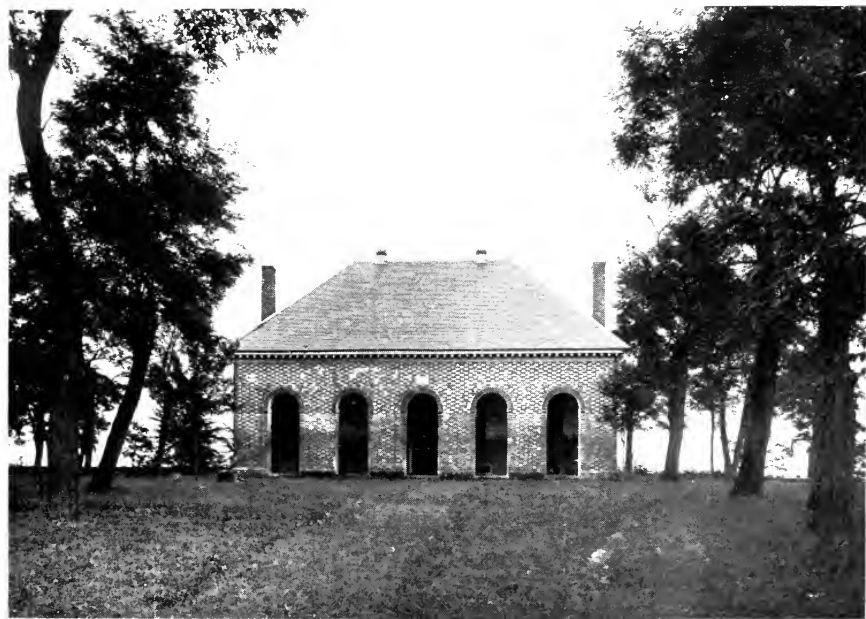
HANOVER COURT HOUSE, VIRGINIA
