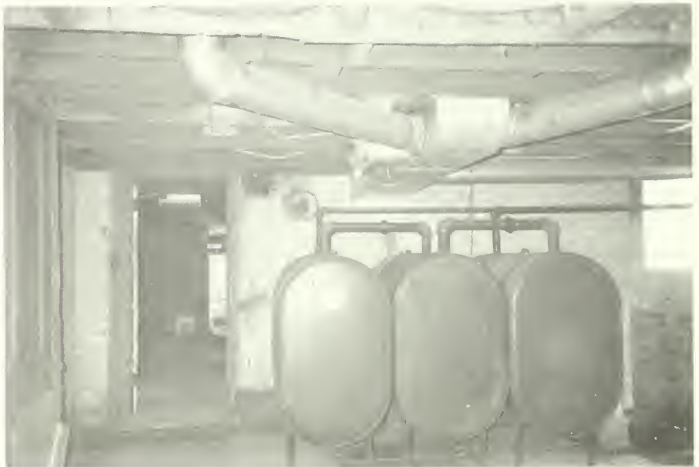
Photo E-68 View looking west in room B05. Moorhead Cottage 1992
