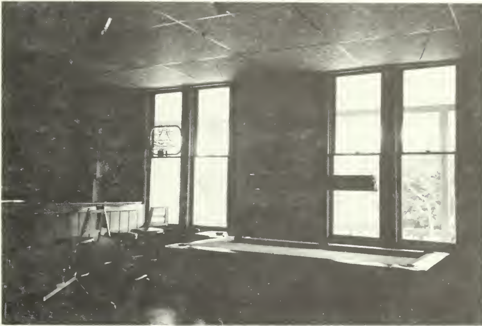
o E-14 East wall of current bar, room 102. Clubhouse 1992
