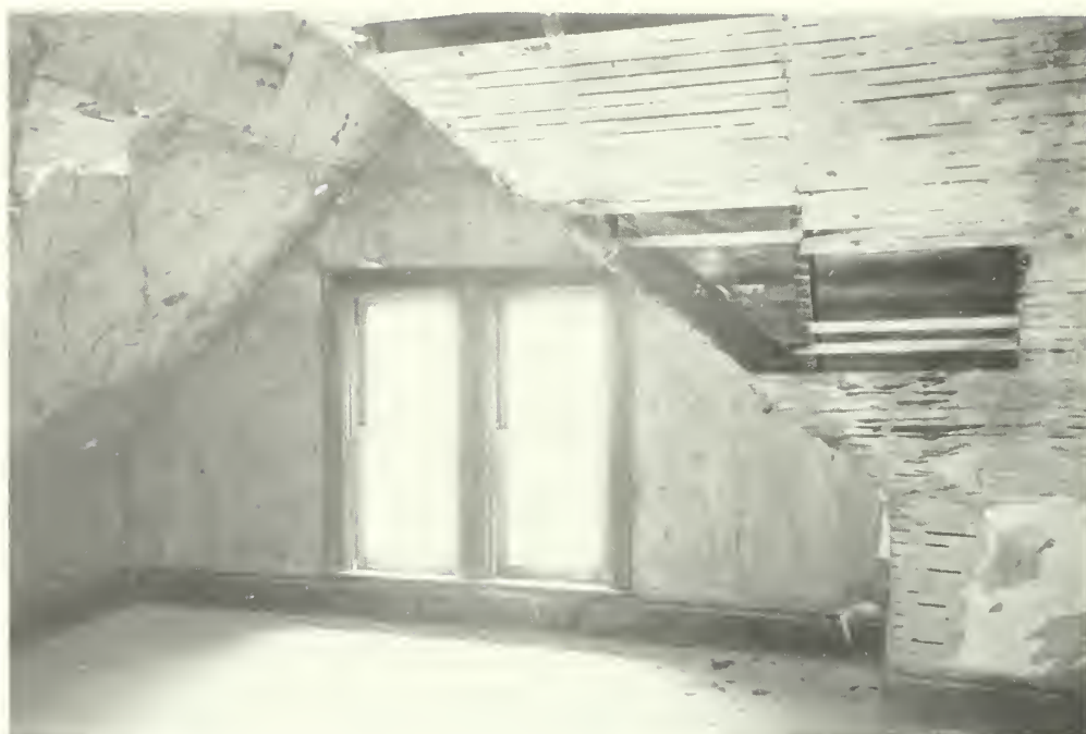
Photo E-55 South wall of room 302. Brown Cottage 1992
