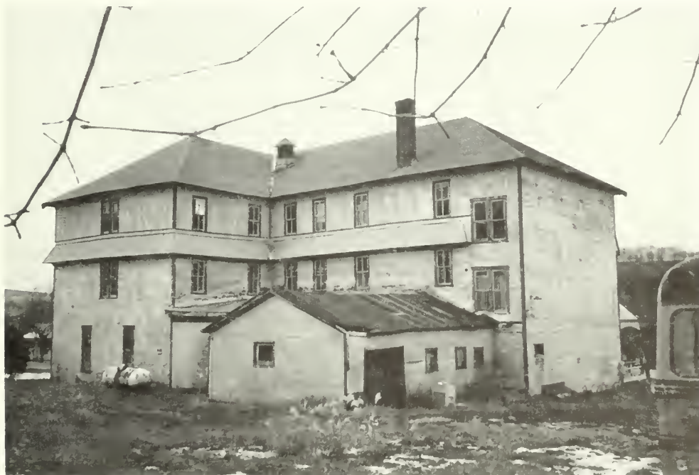
E-12 View of west and south elevations. Clubhouse 1992
