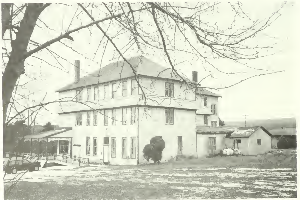
Photo E-10 View of north and west elevations. Clubhouse 1992
