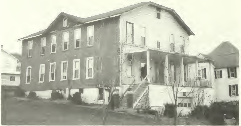
Photo E-94 South and east elevations. Clubhouse Annex 1992
