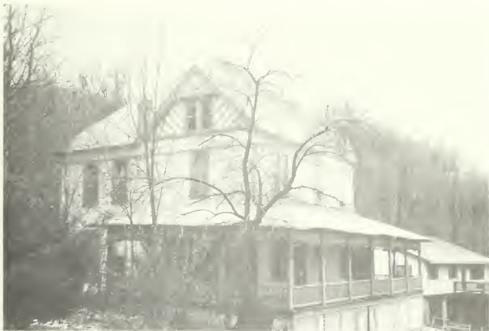
E-34 View of south and east elevations. Brown Cottage 1992
