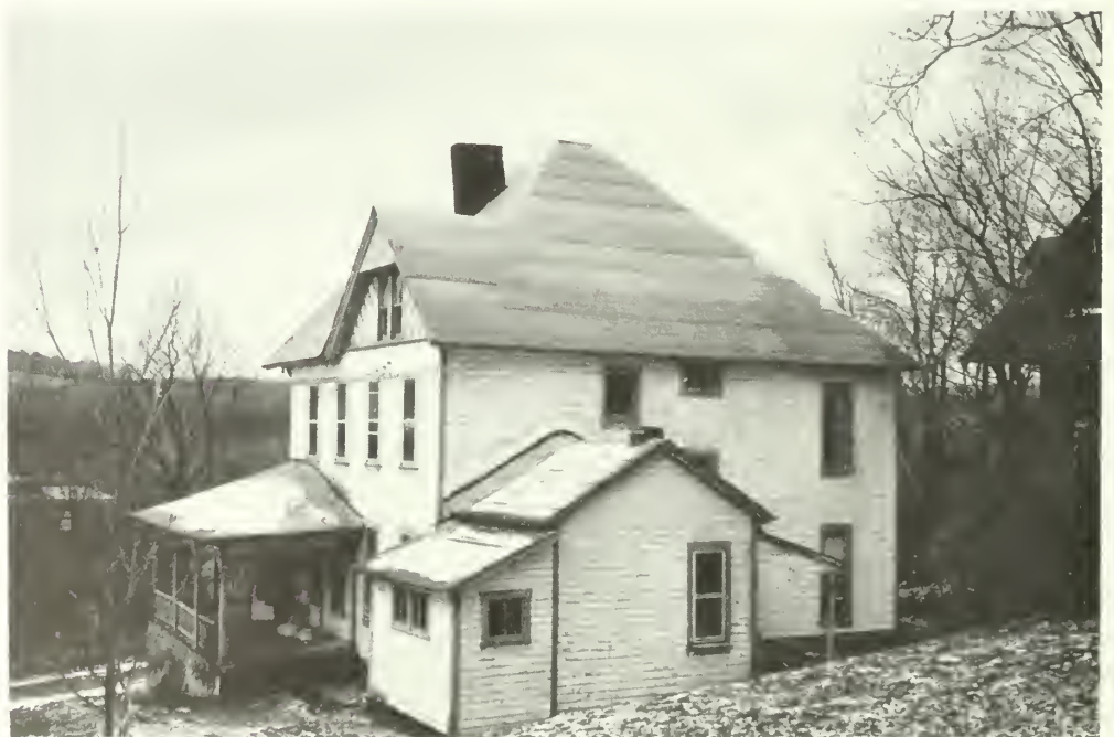
Photo E-33 View of north and west elevations. Brown Cottage 1992
