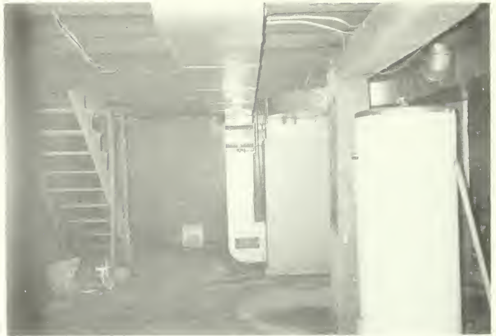
Photo E-67 View looking west in room B04. Moorhead Cottage 1992
