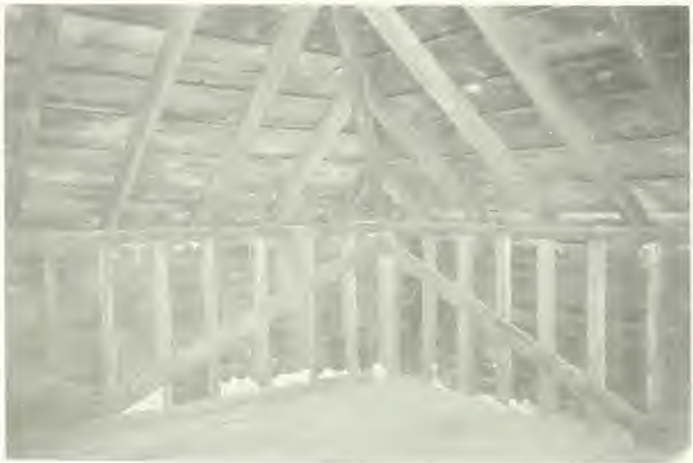
Photo E-93 Southwest corner of attic space 303. Moorhead Cottage 1992
