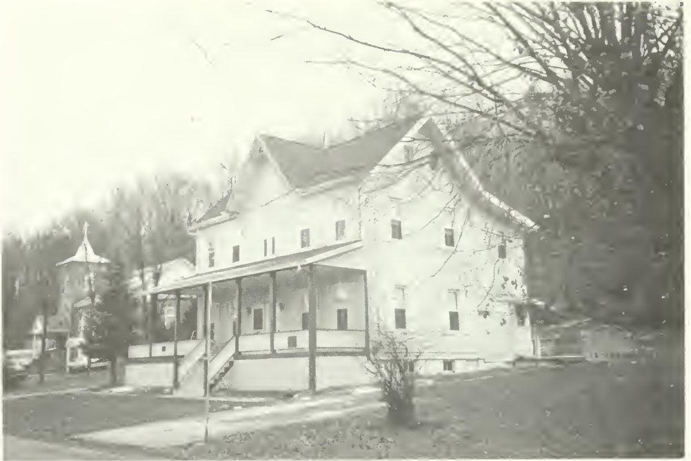
Photo E-5 View looking southwest towards Cottage No. 9. 1992
