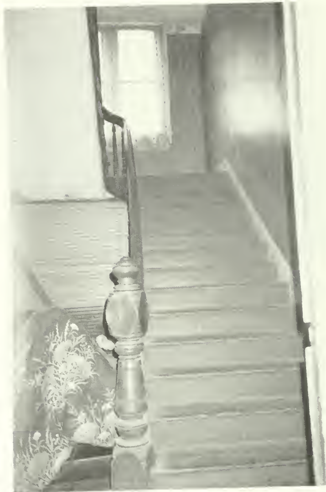
Photo E-13 First floor south stair (room 100) looking west. Clubhouse 1992
