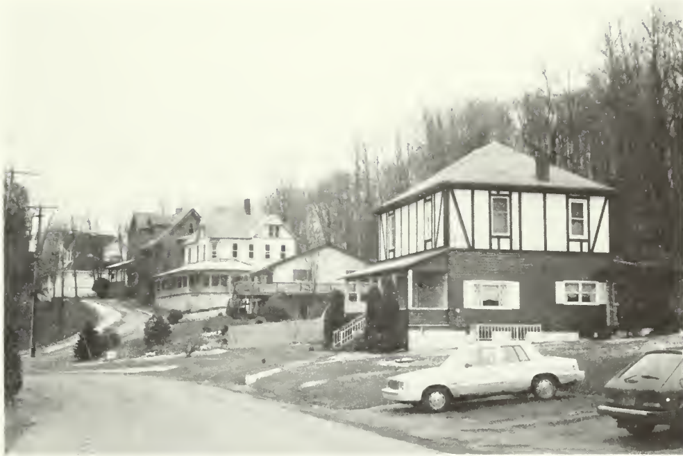
Photo E-3 Looking south past the heavily remodeled Cottage No. 6 in the foreground, and the site of Cottage No. 5, to Cottages Nos. 4, 3, and 2 in the background. 1992
