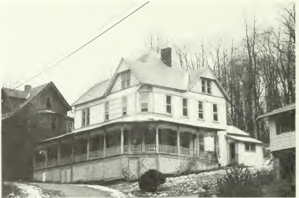
Photo E-32 View of east and north elevations. Brown Cottage 1992
