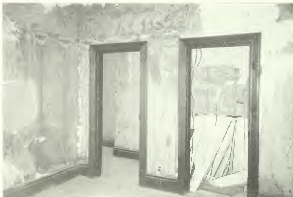
Photo E-56 Northwest corner of room 302. Ghost of former doorway is faintly visible in wall in hallway beyond left doorway. Brown Cottage 1992
