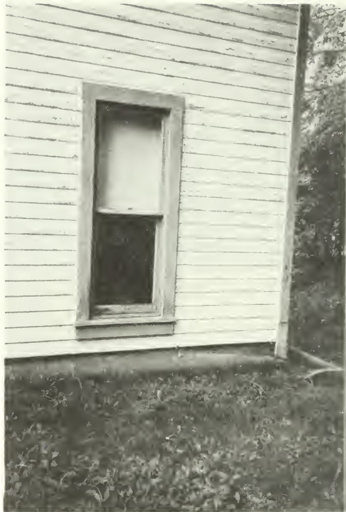
Photo E-36 View of west wall and concrete foundation. Brown Cottage 1992
