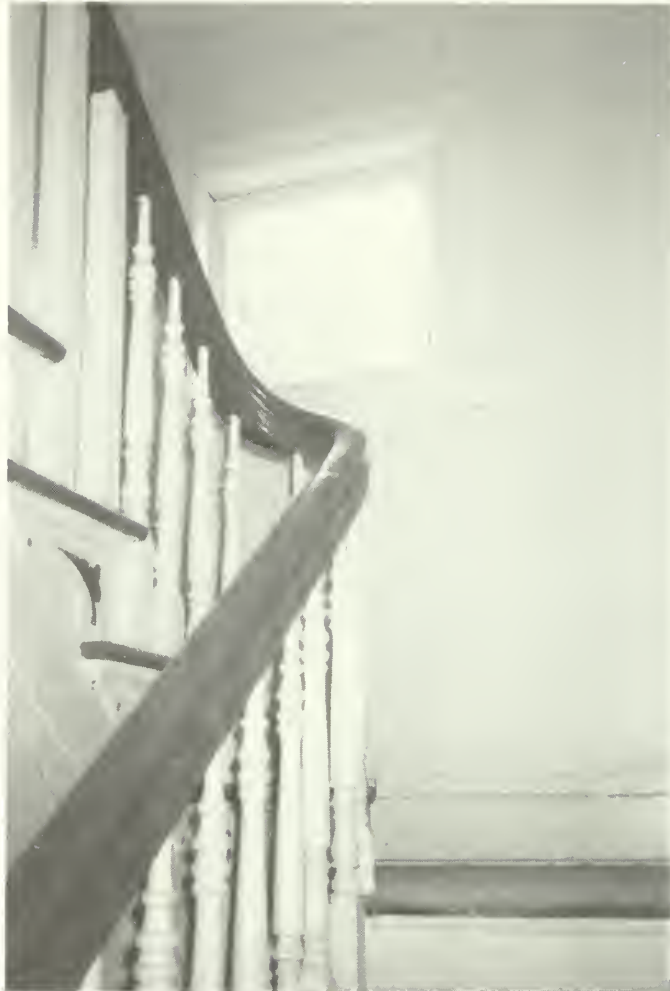
Photo E-46 Detail of change in spindle style in stair at landing between first and second floors in room 100. Brown Cottage 1992
