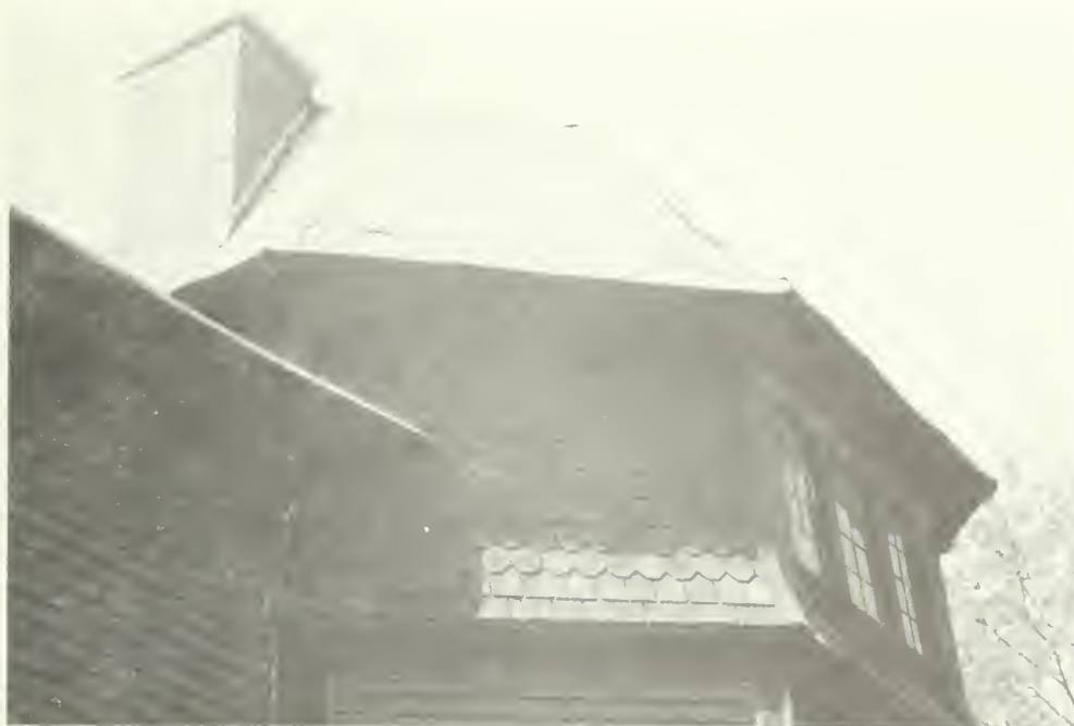
E-65 View of southwest wall of tower showing original wood shingles at third floor. Moorhead Cottage 1992
