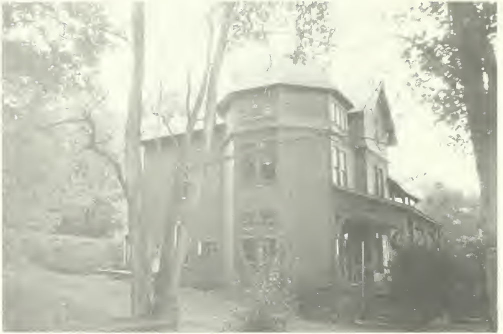
Photo E-1 South elevation of Cottage No. 3 (Moorhead). 1992
