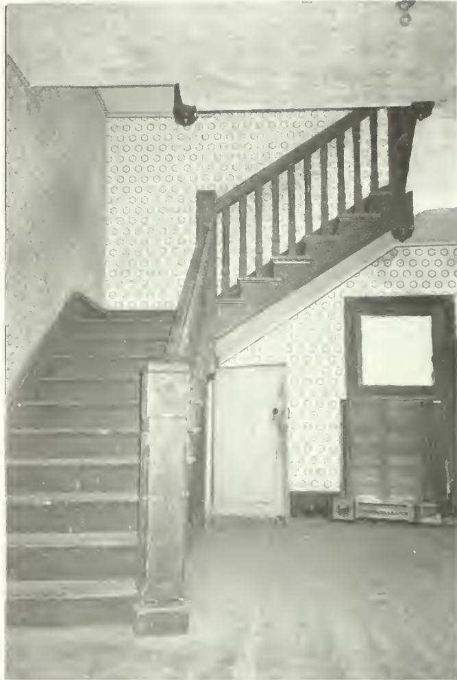
Photo E-71 Looking west in room 100 to main staircase. Moorhead Cottage 1992
