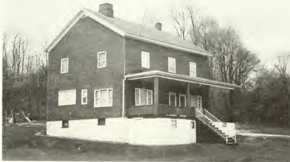
Photo E-8 View looking northwest towards Cottage No. 14. 1992
