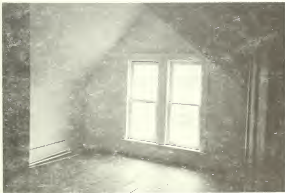
E-59 View of northwest corner in room 304. Brown Cottage 1992
