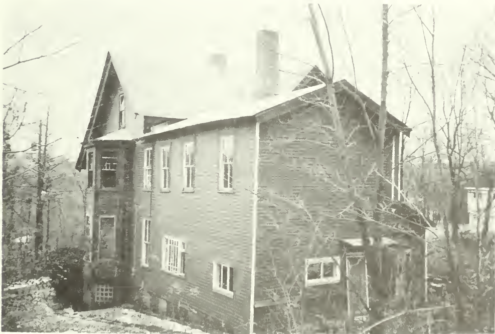
E-63 North elevation and partial west elevation. Moorhead Cottage 1992
