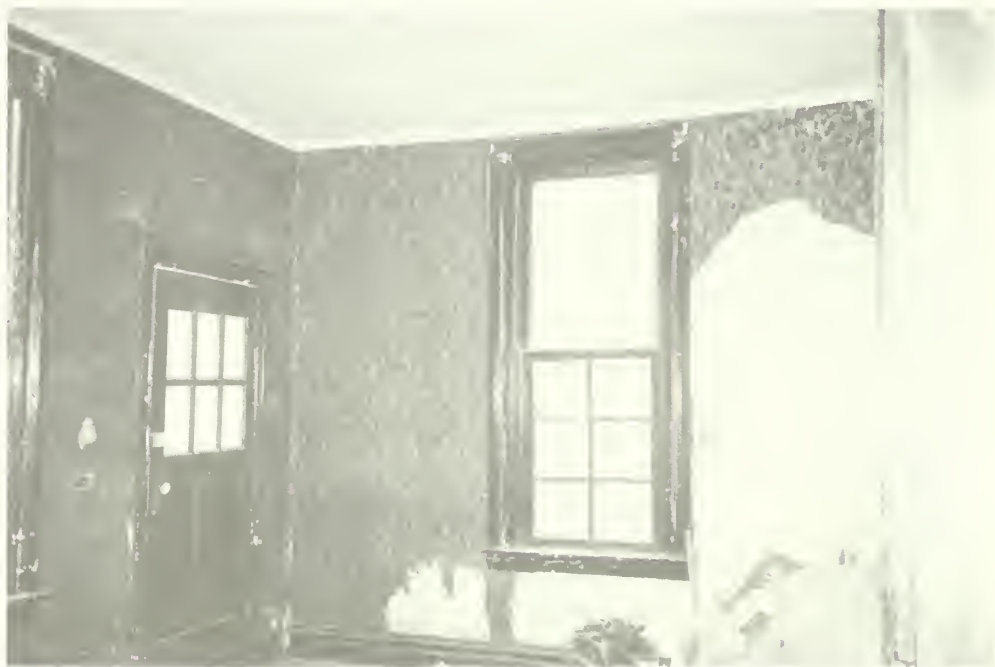
Photo E-75 Southwest view of room 103 showing window and door alterations. Moorhead Cottage 1992
