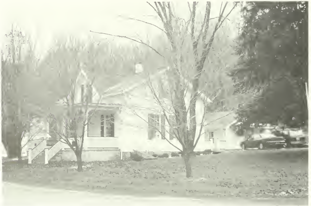
Photo E-6 View looking southwest towards Cottage No. 10. 1992
