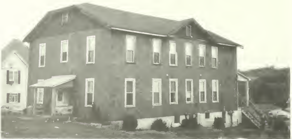
Photo E-95 West and south elevations. Clubhouse Annex 1992
