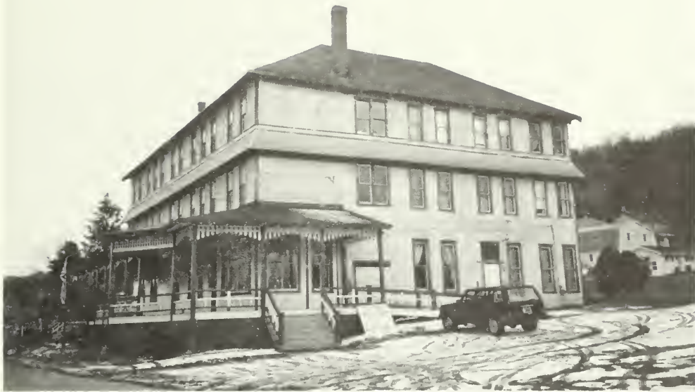
E-11 View of east and north elevations. Clubhouse 1992
