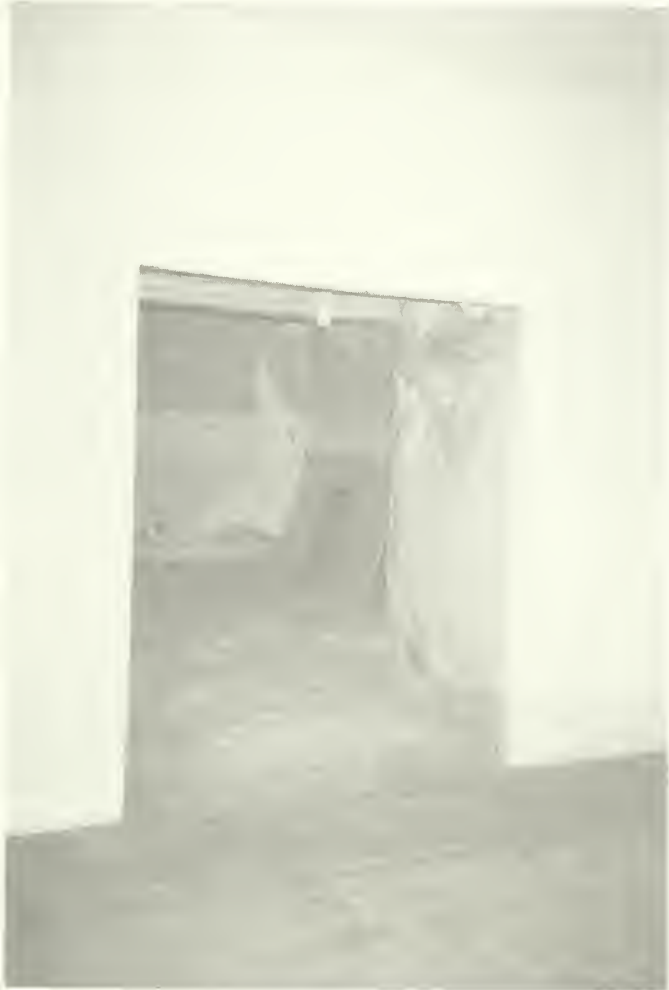
Photo E-40 West wall of room 105 looking into room 103. Brown Cottage 1992
