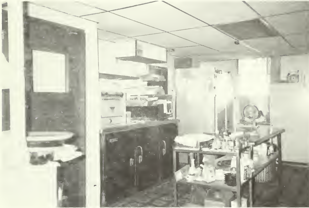
to E-21 Existing first floor kitchen in room 107, looking northeast. Clubhouse 1992
