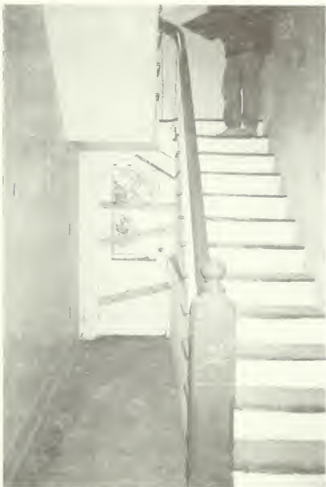
Photo E-45 West view of stair and hall, room 100. Brown Cottage 1992
