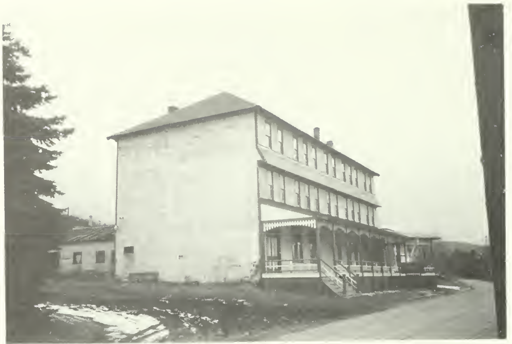
Photo E-9 View of east and south elevations. Clubhouse 1992
