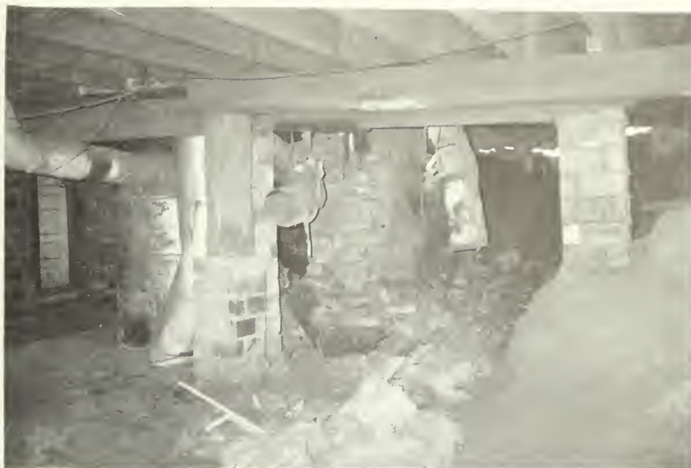
E-69 View looking southeast in room B01. Moorhead Cottage 1992
