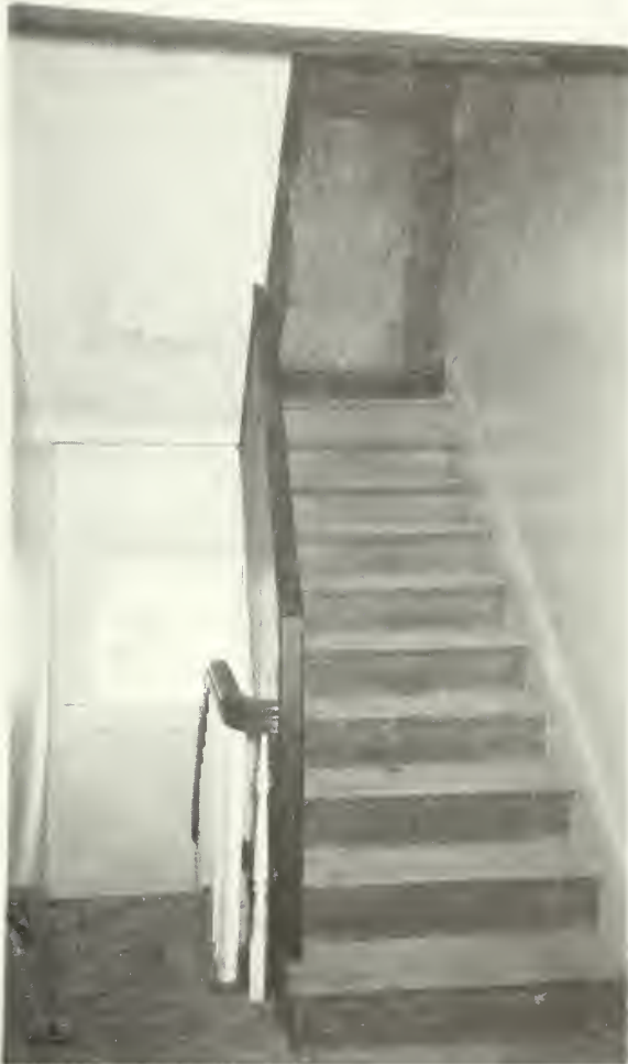
Photo E-47 Second floor view of the main stair from the hall (room 200), looking west. Brown Cottage 1992
