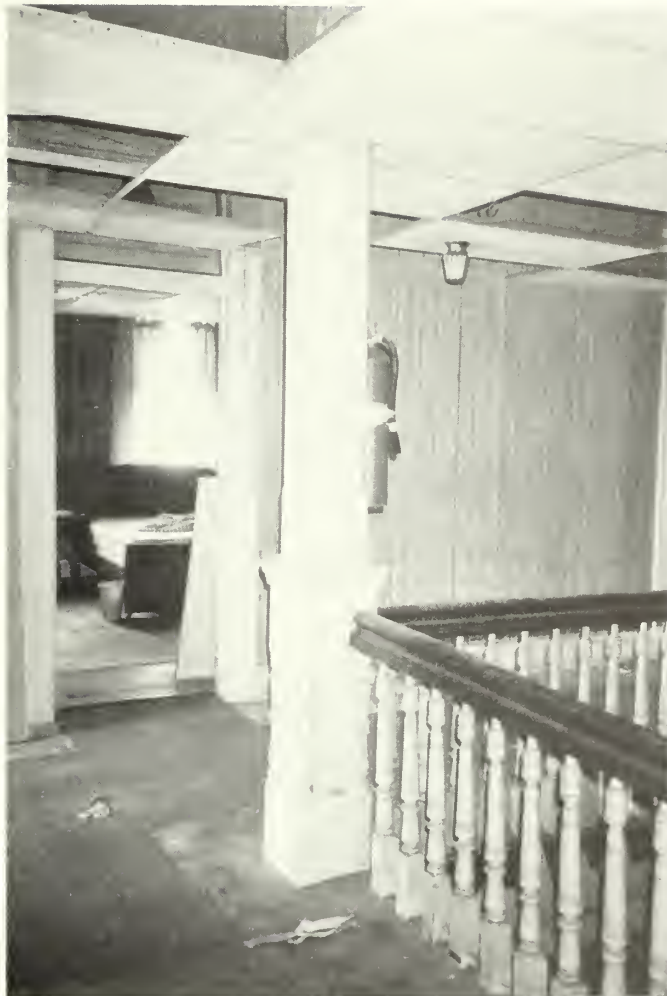
Photo E-30 Third floor hall and main stair looking east. Clubhouse 1992
