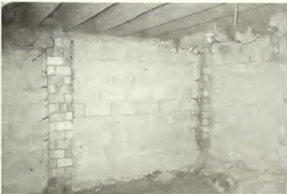
E-70 Northeast corner of room B01 indicating masonry pier and infill structural system. Moorhead Cottage 1992
