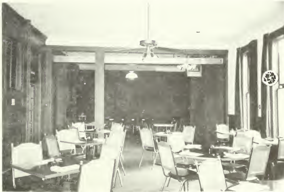
to E-22 Looking west from room 109 into room 113. The off-centered column was originally enclosed in a wall dividing these two rooms. Clubhouse 1992.
