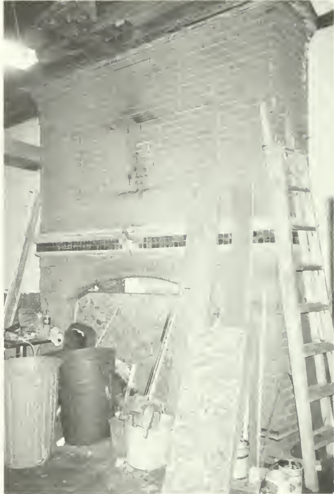
Photo E-16 View of fireplace on west wall of room 106. Clubhouse 1992
