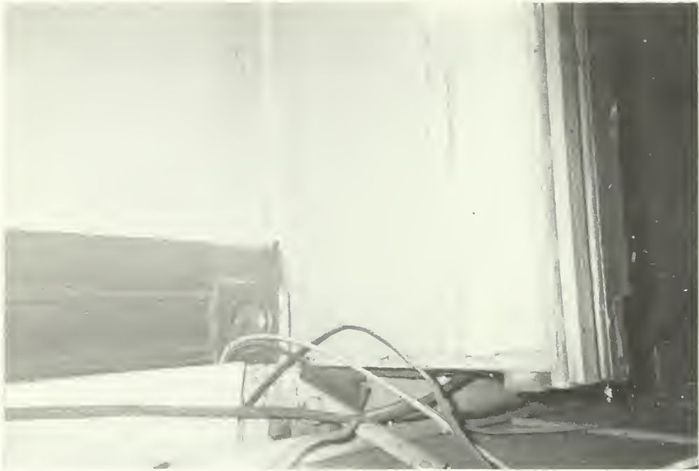
Photo E-19 View looking southwest above existing ceiling in room 107, showing original hall wall and upper part of door which once connected room to west. The door trim with the rose blocks in the south wall is later. Clubhouse 1992
