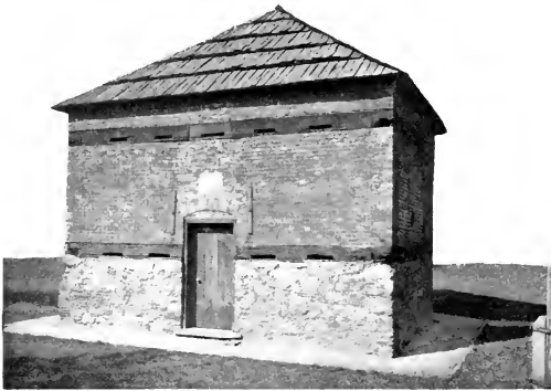
BLOCKHOUSE OF FORT PITT. BUILT IN 1764.
