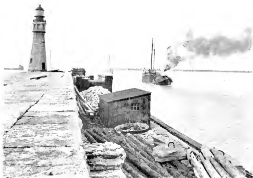
BEACON ON OLD BREAKWATER.
