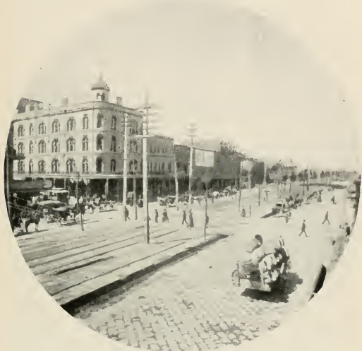
CANAL STREET, NEW ORLEANS.
