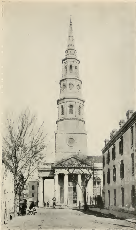
ST. PHILIP'S CHURCH, CHARLESTON.
