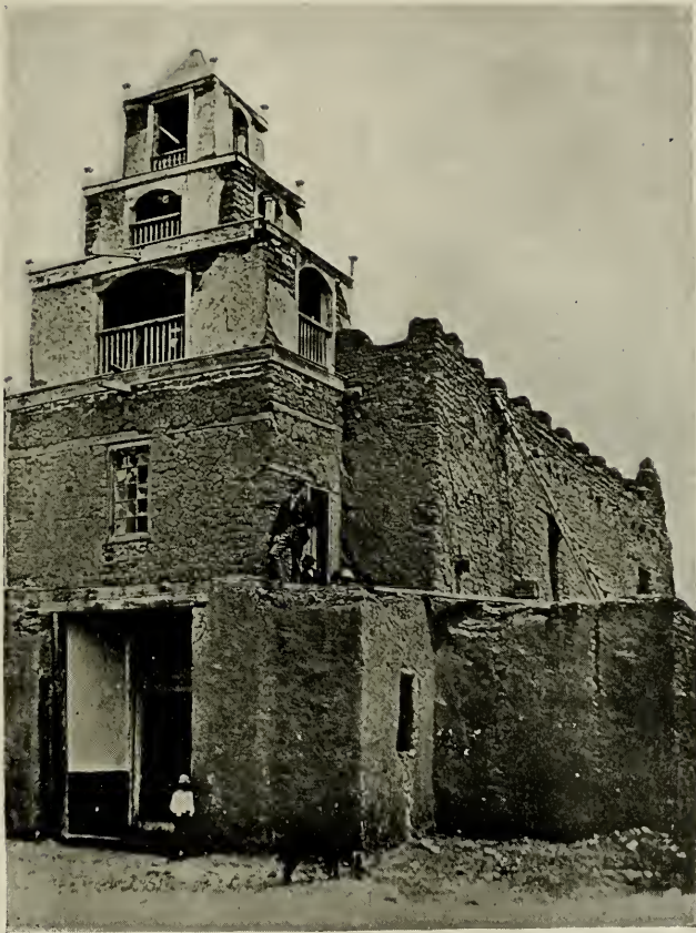
SAN MIGUEL CHAPEL BEFORE RECONSTRUCTION.
