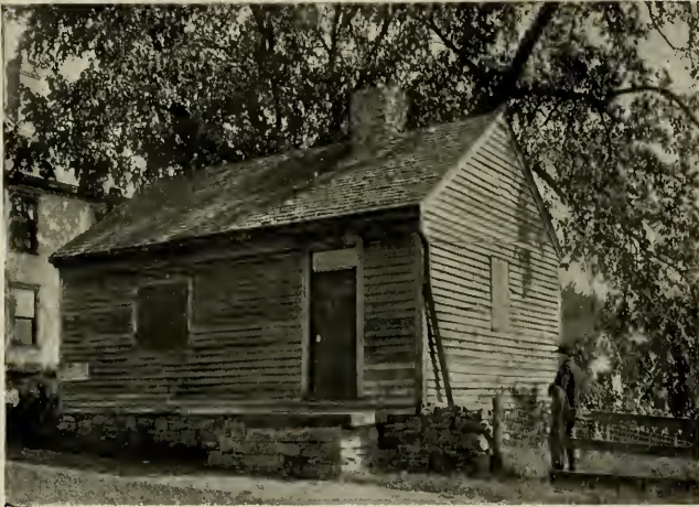
OHIO COMPANY'S LAND OFFICE.
