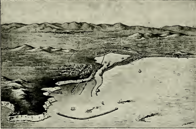
IMPROVED HARBOR OF SAN PEDRO, PORT OF LOS ANGELES.
