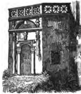
PORCH AT CHELVY COURT HOUSE.
