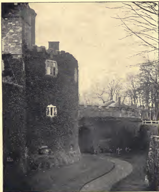
Bridge across Moat.
