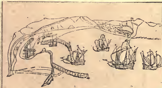
The town, castle, and harbour of Dover in the time of Henry VIII.
