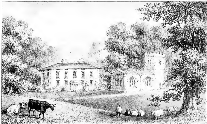
THE HOUSE AT ST. JOHN'S
