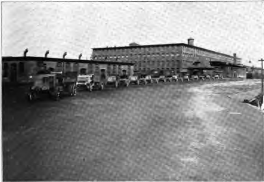
PLANT OF THE LOCOMOBILE COMPANY OF AMERICA, BRIDGEPORT
