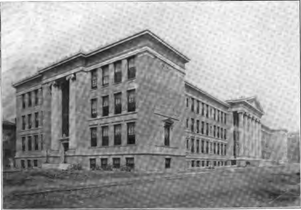
NEW HIGH SCHOOL BUILDING, BRIDGEPORT
