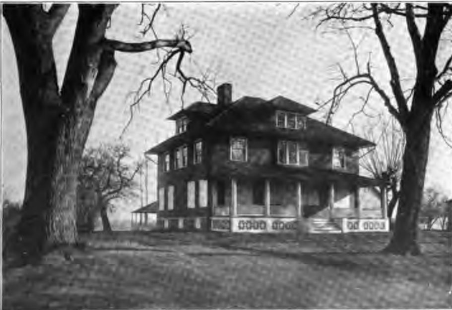
FAIRFIELD FRESH AIR HOME FOR CHILDREN
