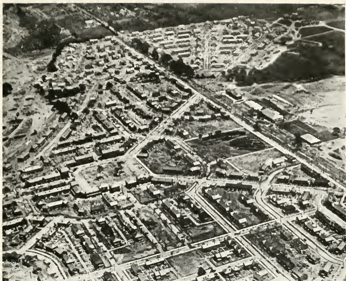
FAIRVIEW, FORMERLY CALLED YORKSHIP VILLAGE A part of the war-time housing development undertaken in cooperation with the Emergency Fleet Corporation.
