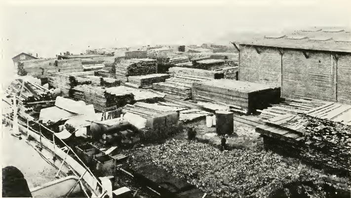
LUMBER YARD AT NORTH END OF PLANT
