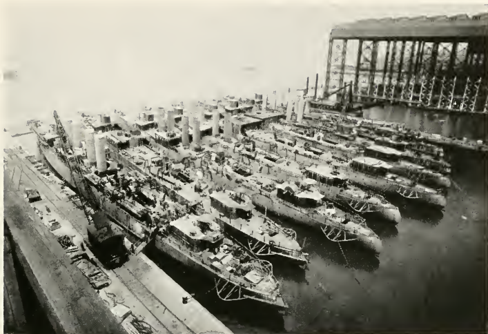
A GROUP OF DESTROYERS BEING OUTFITTED IN ONE OF THE WET BASINS
