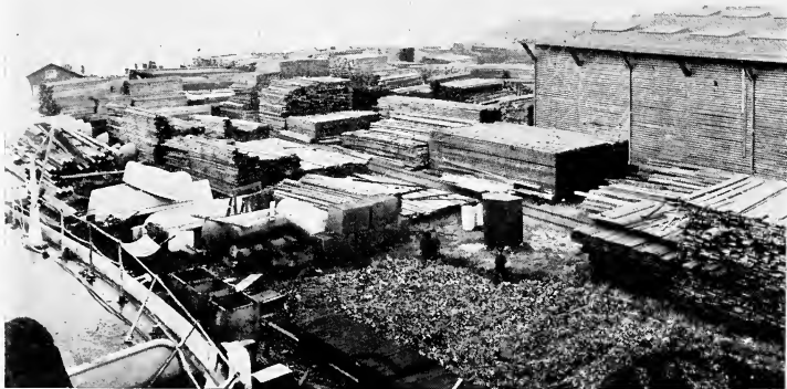
LUMBER YARD AT NORTH END OF PLANT
