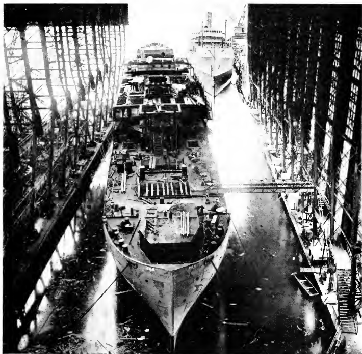
PASSENGER LINERS OUTFITTING IN THE WET SLIP
