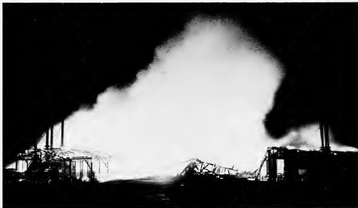
PLATE AND ANGLE SHOP BEHIND DESTROYER WAYS, BURNED SEPTEMBER 11, 1918
