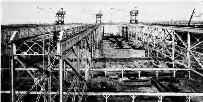
THE FIRST KEELS BEING LAID ON THE SOUTH YARD WAYS
