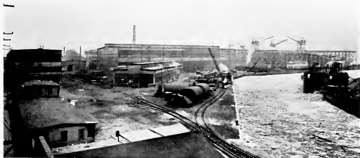
SOUTH YARD SHOP AND WAYS
