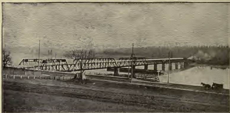
FRASER RIVER BRIDGE, NEW WESTMINSTER.
