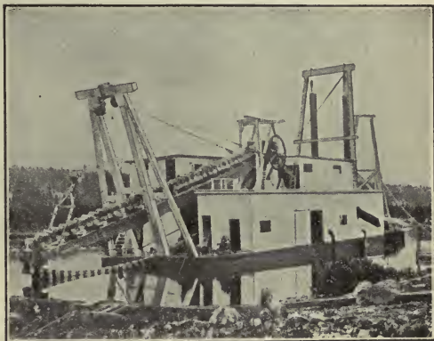
DREDGE AT GOLD RUN.
