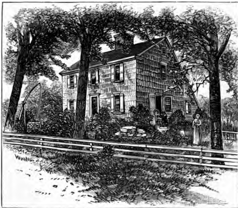
HOUSE NEAR GREENFIELD HILL, TOWN OF FAIRFIELD, FAIRFIELD COUNTY, CONNECTICUT, BUILT BY GERSHOM HUBBELL IN 1751. STANDING IN 1881.
