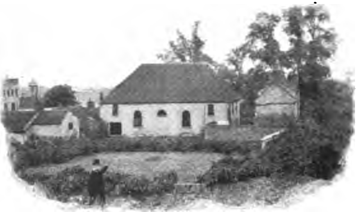
OLD KINGSWOOD, FROM THE NORTH.
