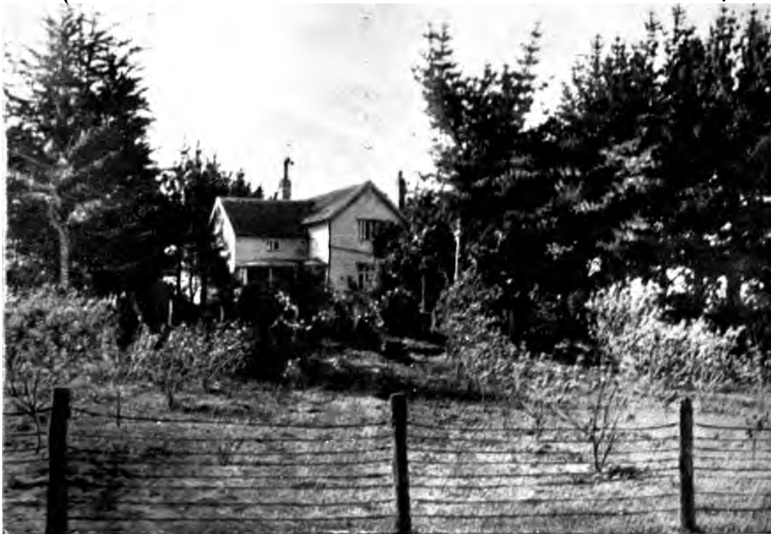
PRINCIPAL'S RESIDENCE, THREE KINGS COLLEGE.
