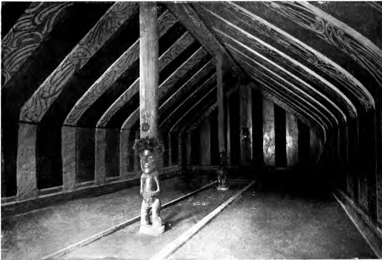
WHAREPUNI AT KORINITI (CORINTH) WANGANUI RIVER.
