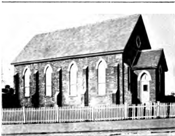
HOBSON STREET CHURCH.
