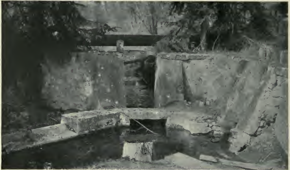
German Concrete Strong Point in the Dam near Chateau Diable.
