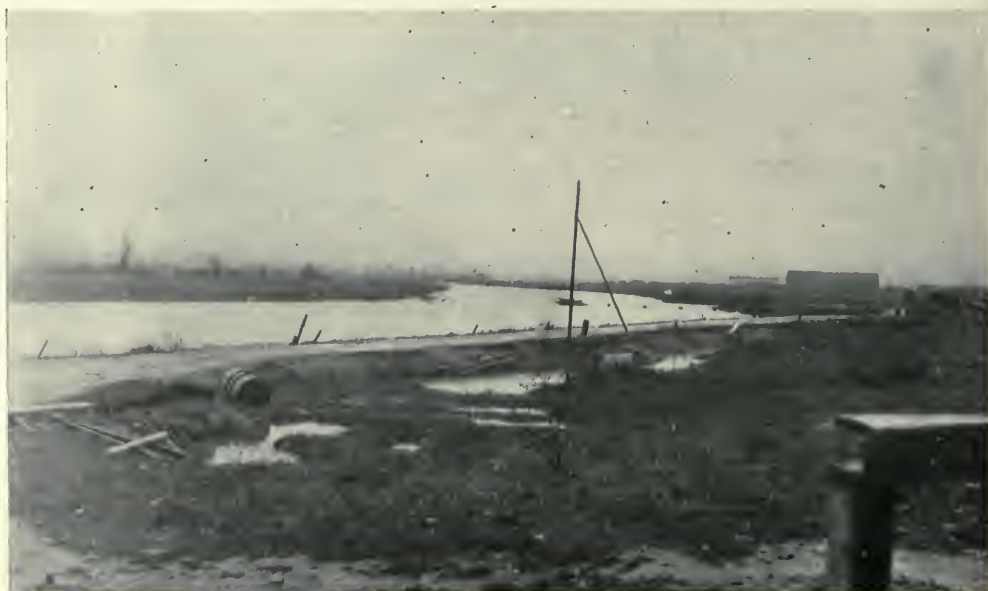
Journey's End. Piles in river indicate probable position of engineer bridge at Villers-devant-Mouzon, over which a platoon of K Company crossed—the first unit of the 77th Div. to establish a position on the far side of the Meuse River.
