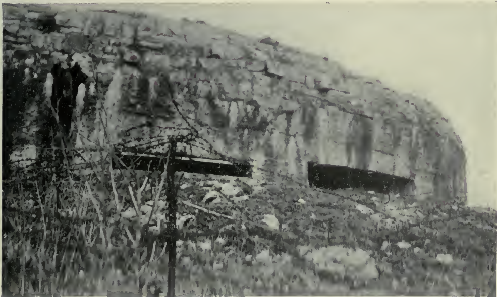
Portion of German Emplacement, a Large “Pill Box,” at Domèvre.
