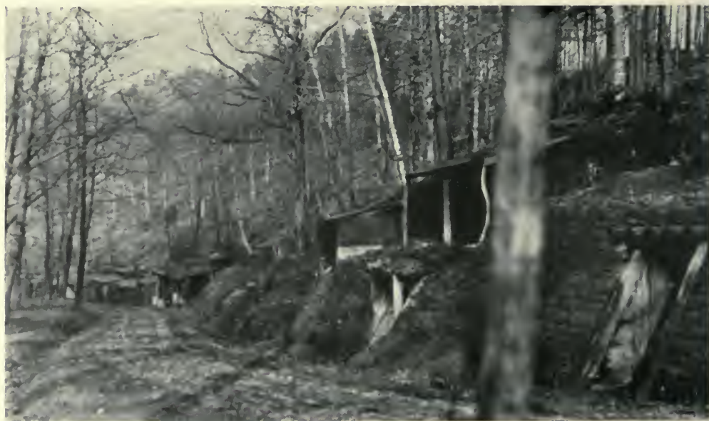
French Kitchens and Bomb-Proofs at Nouveau Cottage.
