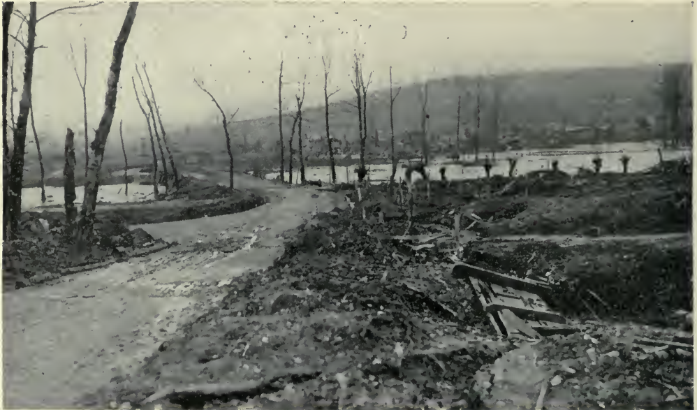
Reconstructed Bridge Over Vesle Between St. Thibaut and Bazoches, and Formidable Heights to the North.
