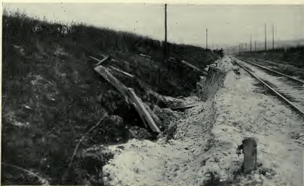
A Defensive Position Was Dug in the Railroad Bank West of Bazoches, near La Gravière.
