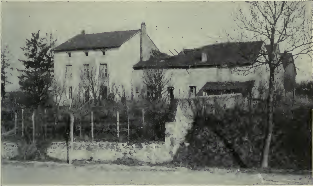
Herberviller—Headquarters of the G. C. "Gainsette."
