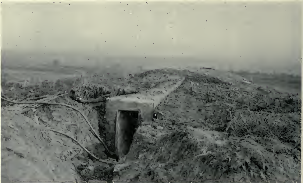
Entrance to German Concrete Machine Gun Emplacement.
