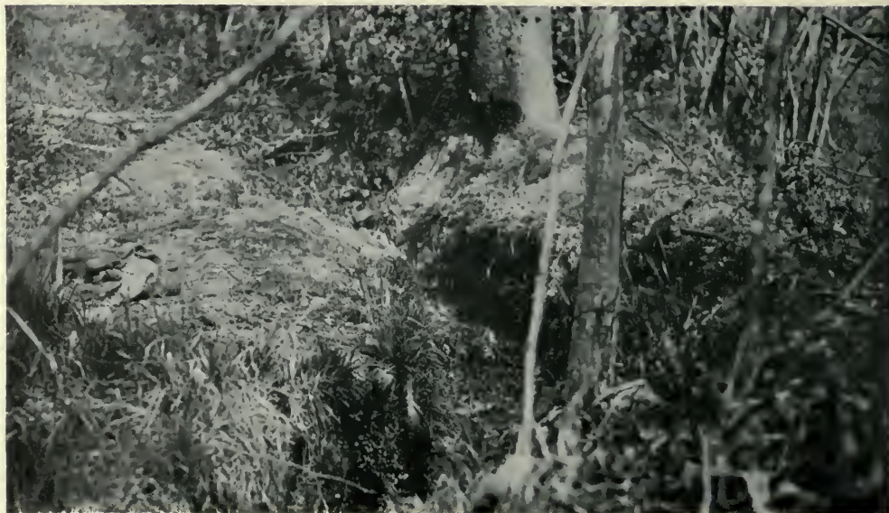
Section of Trench near Chateau Diable.
