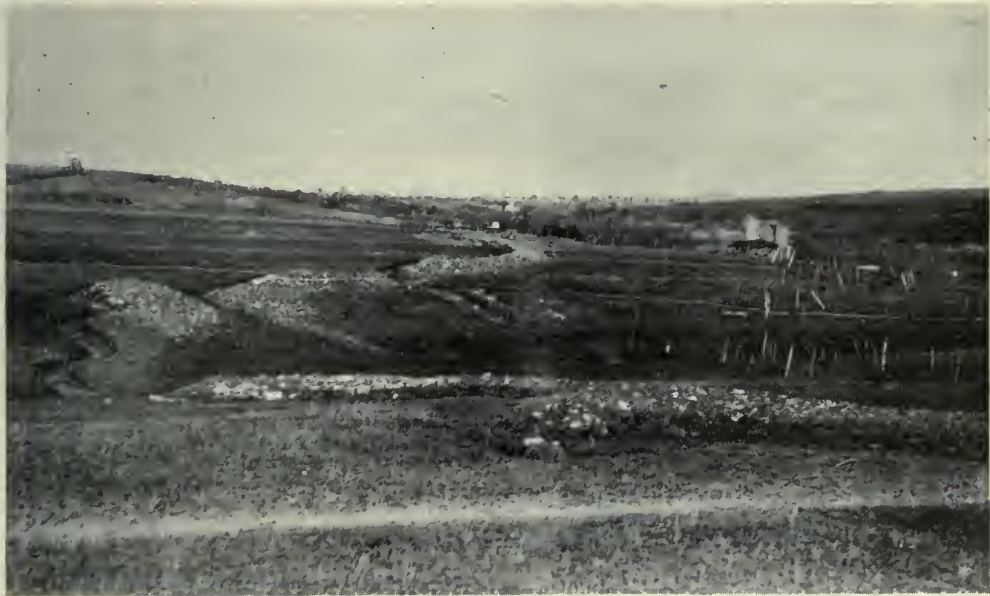
Support Trenches at Pettonville.
