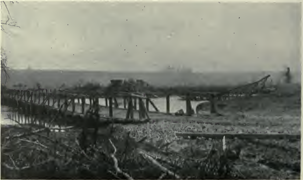
Over this "artillery" bridge, constructed by the 302d Engineers to supplant the one in background, destroyed, our last hot meal was rushed up from Marcq and Martincourt Farm before the jump-off at St. Juvin, Nov. 1.
