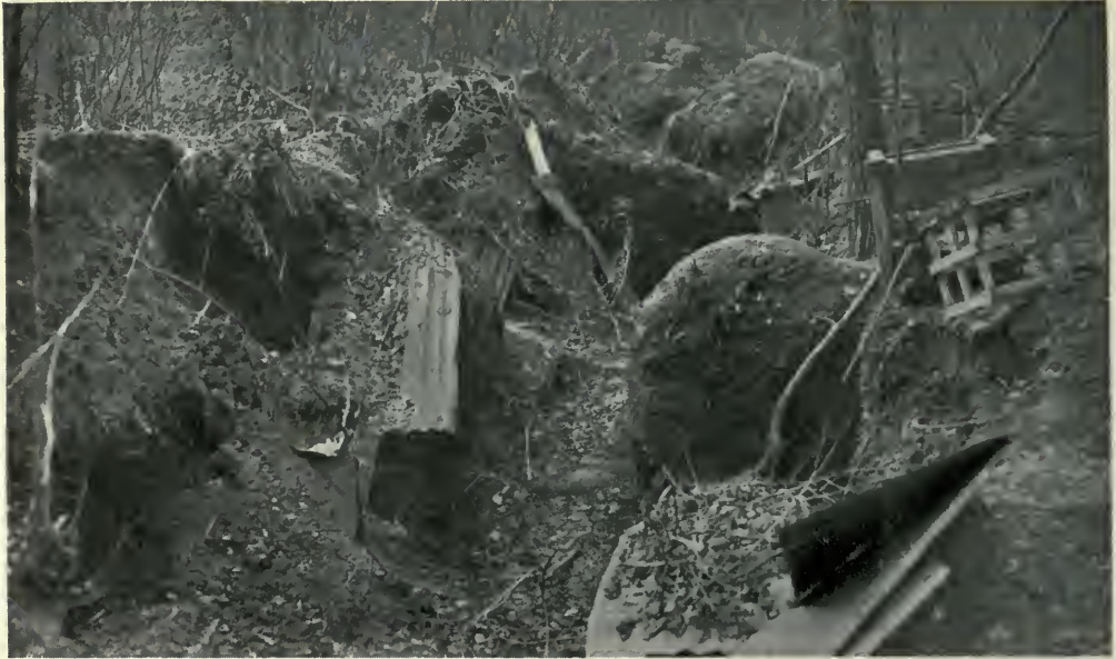
Effects of Shell-fire on Trenches North of Longueval.
