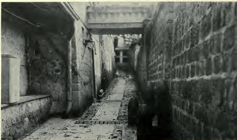
Sunken Entrance to French Commander's Twelve Room P. C.—Nouveau Cottage.
