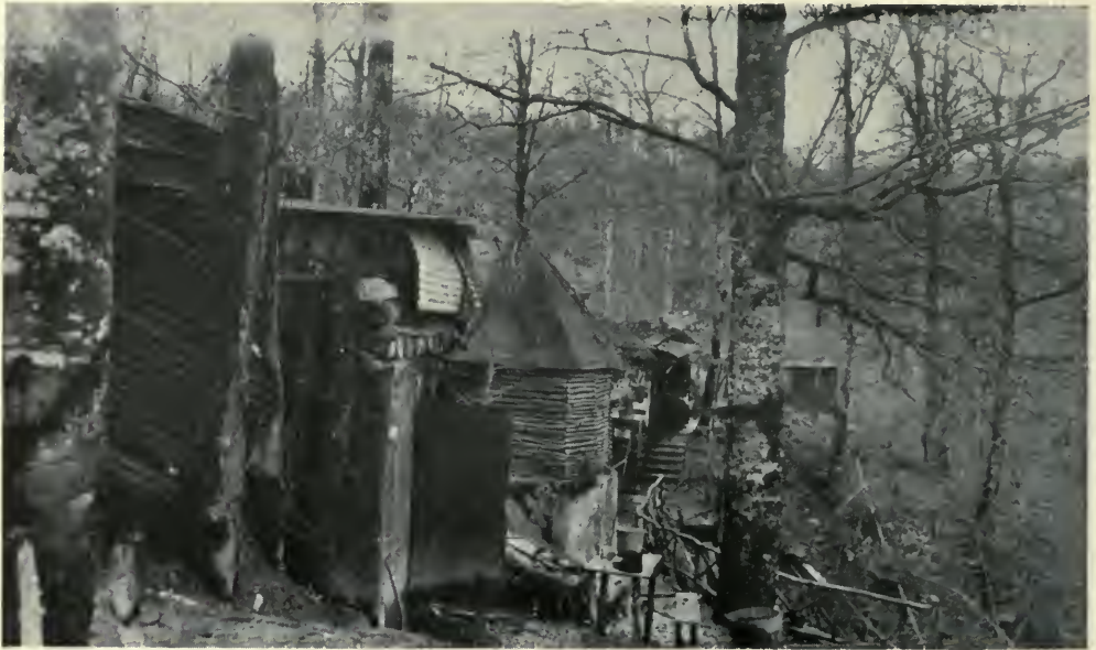
Another View of Concrete German Structures near Abri du Crochet, Occupied by 2nd Bn. When in Reserve.
