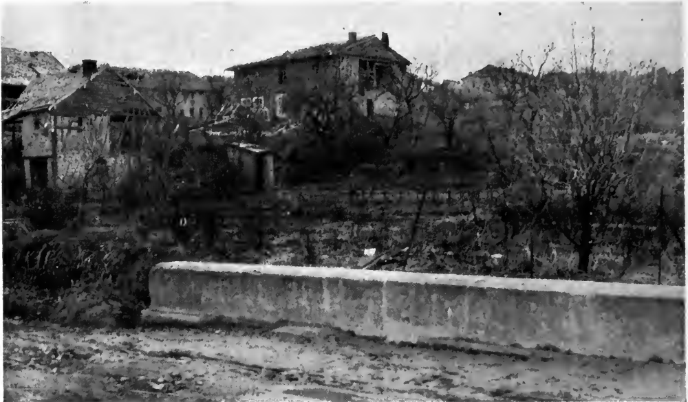
Stone Bridge at East Entrance to St. Juvin, and Graveyard Established Subsequent to the Attack of Nov. 1.
