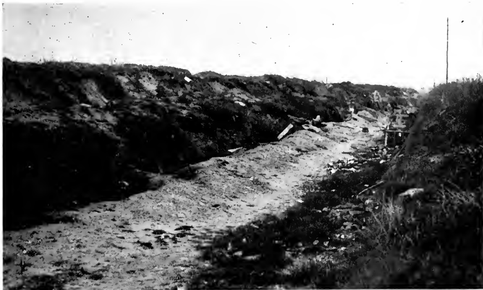
Positions Just Forward of the Railroad Track, West of Bazoches.
