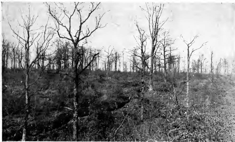
Junction of Boyau Breme and Boyau des Chemis, Looking Northeast.
