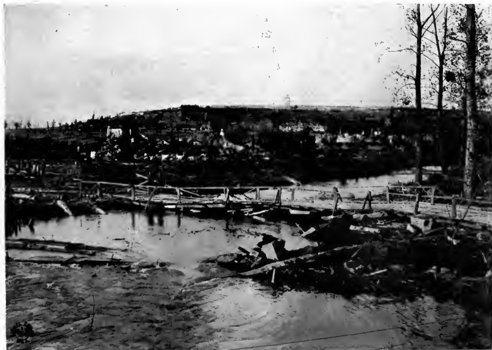
Bridge Hastily Constructed by 302nd Engineers over Vesle River between St. Thibaut and Bazoches.
