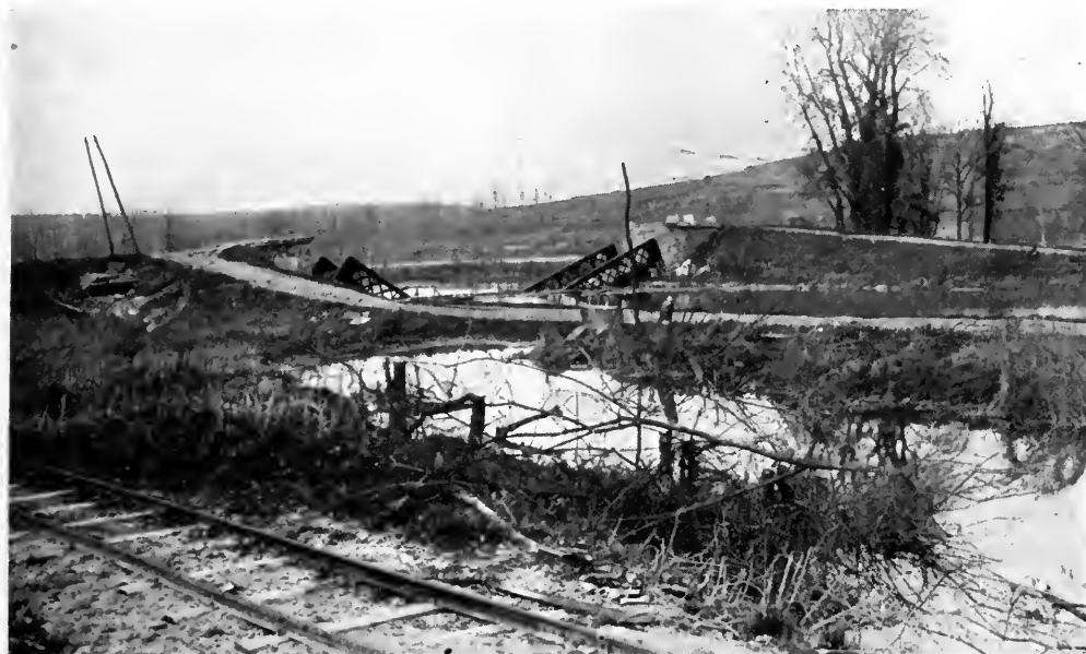
Aisne Canal. During the advance, units of the 1st Bn. saw Germans flee across this bridge, which presently blew up.
