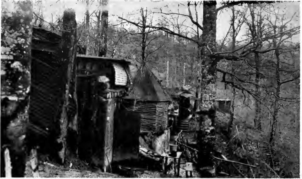
Another View of Concrete German Structures near Abri du Crochet. Occupied by 2nd Bn. When in Reserve.
