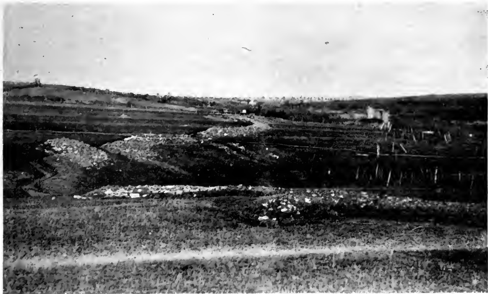
Support Trenches at Pettonville.
