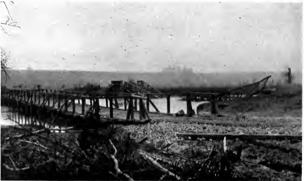
Over this "artillery" bridge, constructed by the 302d Engineers to supplant the one in background, destroyed, our last hot meal was rushed up from Marcq and Martincourt Farm before the jump-off at St. Juvin, Nov. 1.
