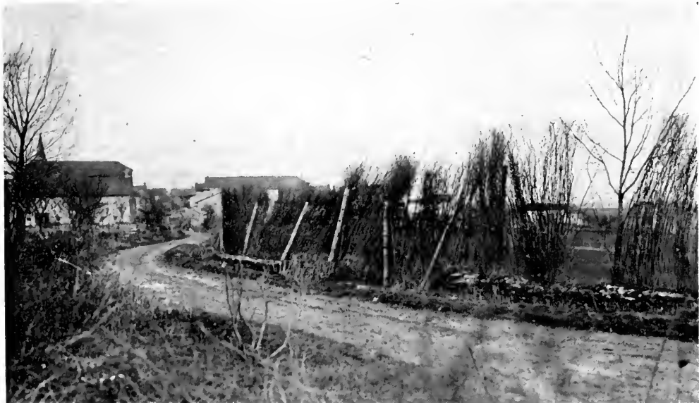
Camouflage at Entrance to Herberviller, on Pettonville Road.
