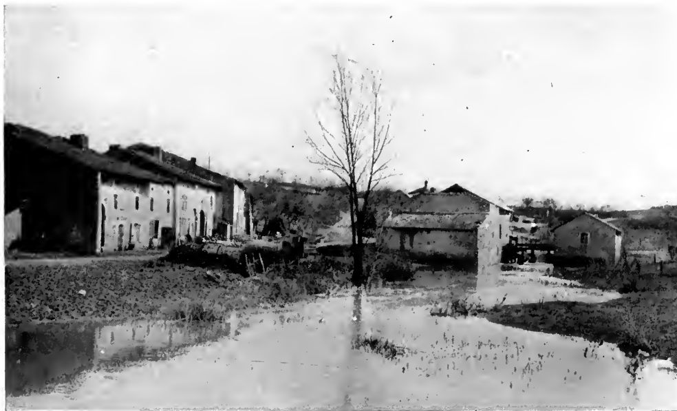
Pettonville—A First-aid Post and Baths Located in the Mill.
