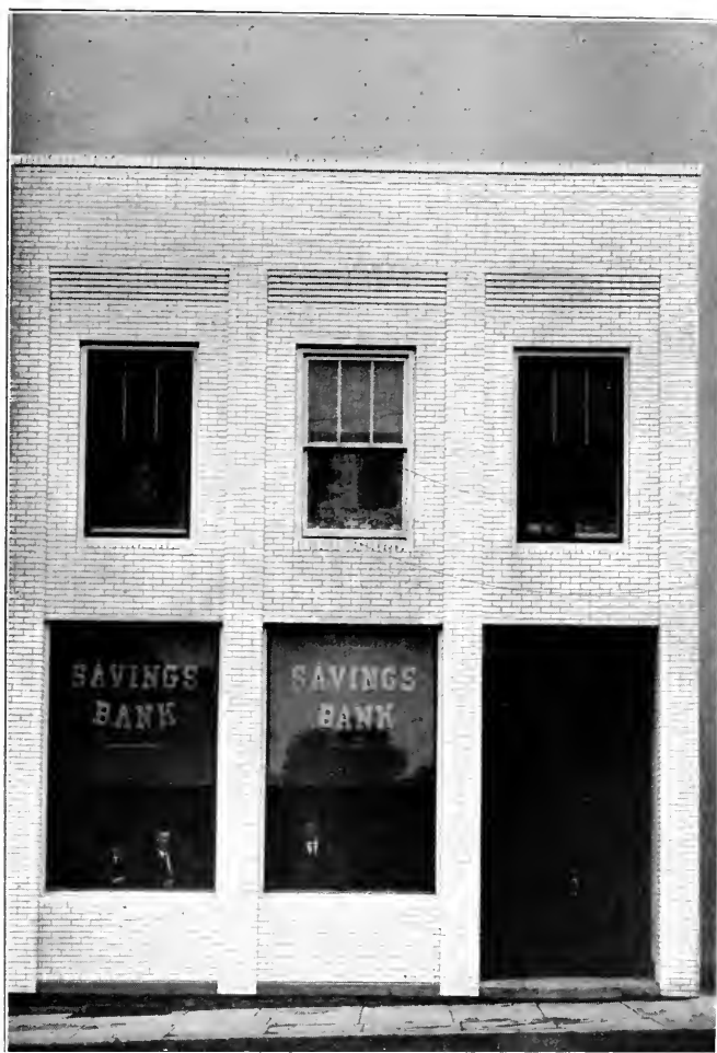
BRIDGEWATER SAVINGS BANK
