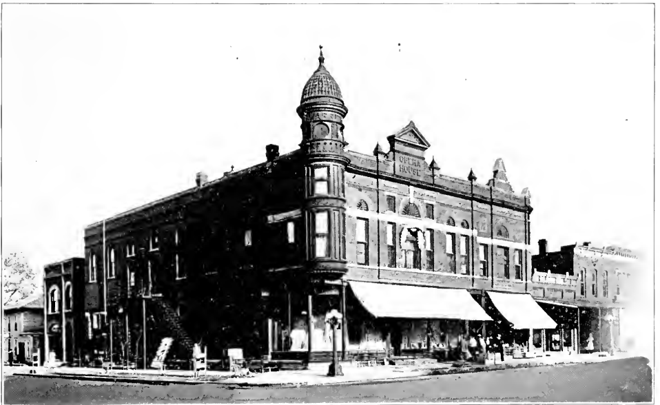
OPERA HOUSE, GREENFIELD
