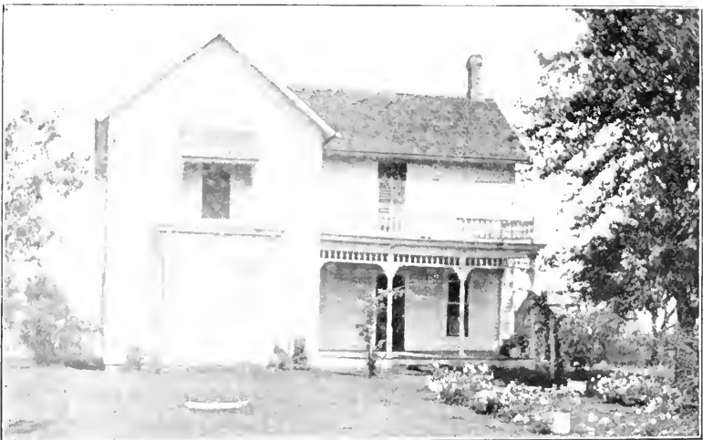
Former Residence of C. H. Wright, near Bullion
