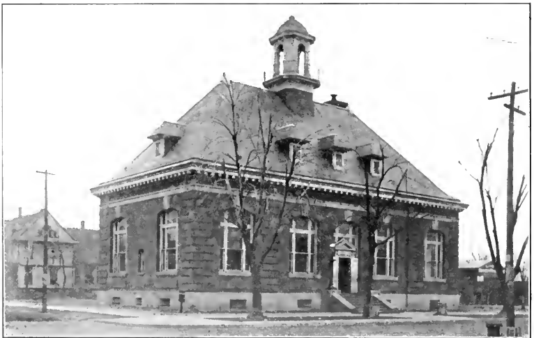
KIRKSVILLE POST OFFICE BUILDING.
