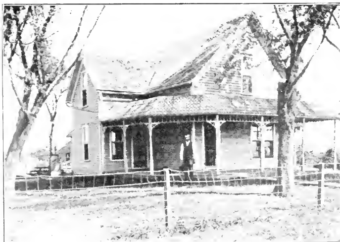
Residence of L. M. Willis, 3 1-2 miles northeast of Kirksville
