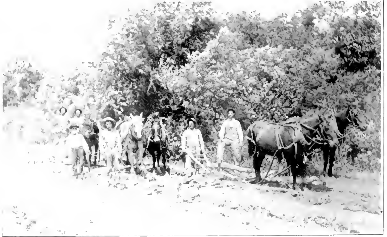
Grant Harless with road grader, near Stahl
