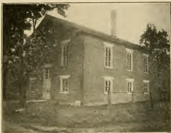
TRINITY LUTHERAN CHURCH, WATERSTREET, PA.
