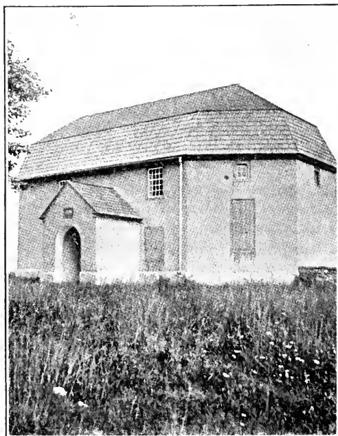
NEW PROVIDENCE CHURCH, BUILT 1743
