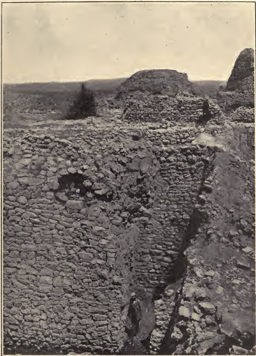
FIG. 4. — Typical wall of the Second City, Troy.
