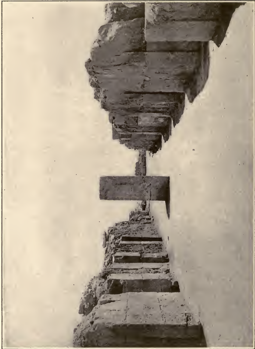
Interior Corridor showing Entrances to Magazines, the Palace, Phaestus.
