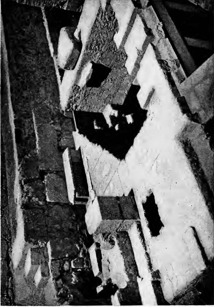
Pavement of Second Floor still in Position, the Palace, Knossos.
