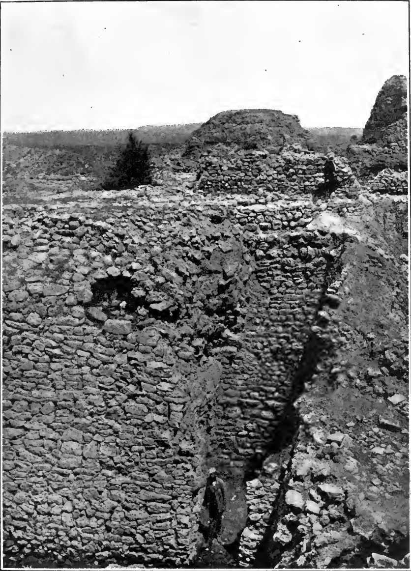
FIG. 4. — Typical wall of the Second City, Troy.
