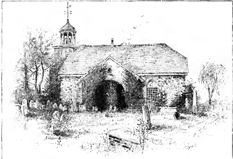
OLD SWEDES' CHURCH, WILMINGTON, DELAWARE.
