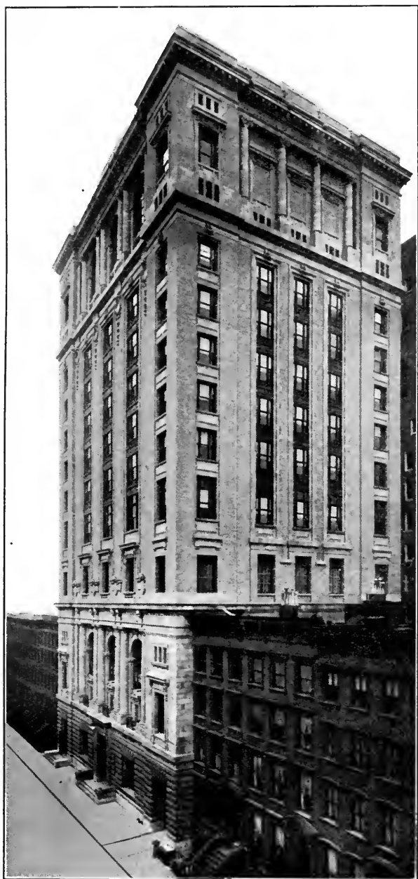
ENGINEERING SOCIETIES' BUILDING, 29 WEST 39TH STREET PRESENT HOME OF THE SOCIETY
