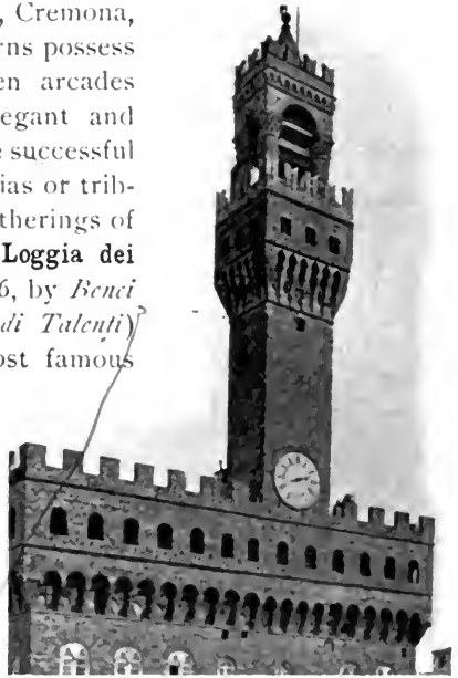
FIG. 155.—UPPER PART OF PALAZZO VECCHIO, FLORENCE.
