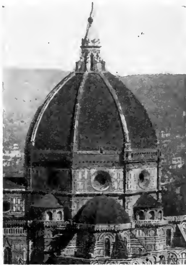
FIG. 160.—EXTERIOR OF DOME OF DUOMO, FLORENCE.
