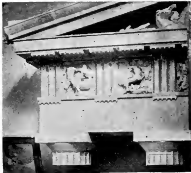
FIG. 27.—DORIC ORDER OF THE PARTHENON.
