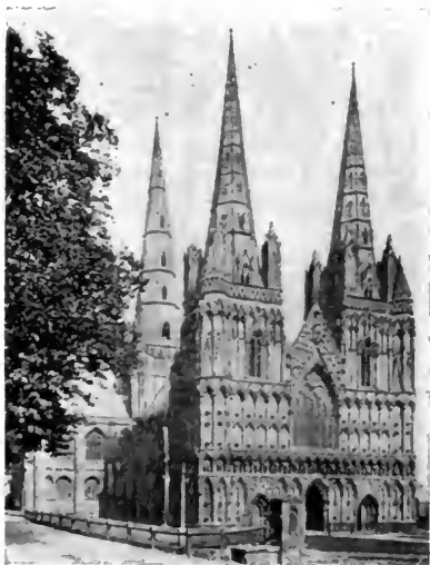
FIG. 134.—WEST FRONT, LICHFIELD CATHEDRAL.
