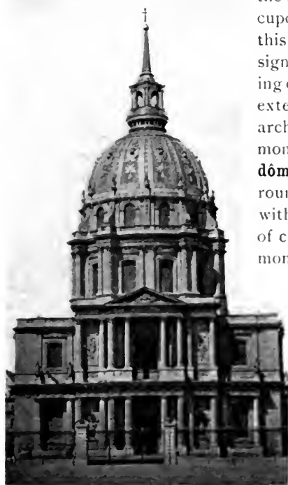
FIG. 182.—DOME OF THE INVALIDES.
