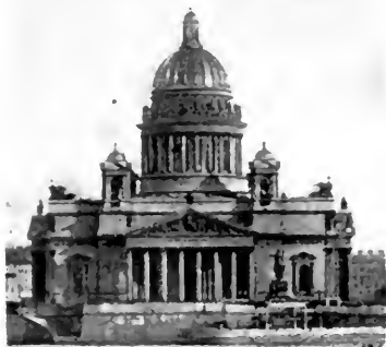
FIG. 207.—ST. ISAAC'S CATHEDRAL, ST. PETERSBURG.
