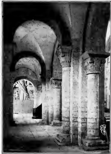
FIG. 134—MORIENVAL. PARISH CHURCH. VIEW OF THE NORTH AISLE
