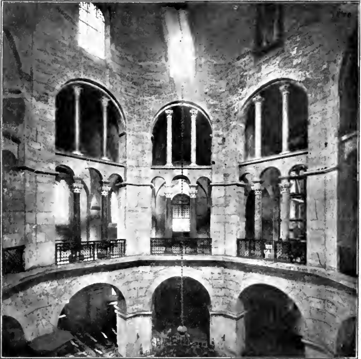
FIG. 85—AIX-LA-CHAPELLE. CHARLEMAGNE'S CHAPEL. INTERIOR
