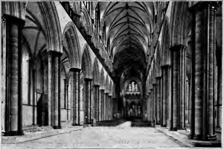
FIG. 157—SALISBURY. INTERIOR OF THE CATHEDRAL, LOOKING TOWARD THE EAST END
