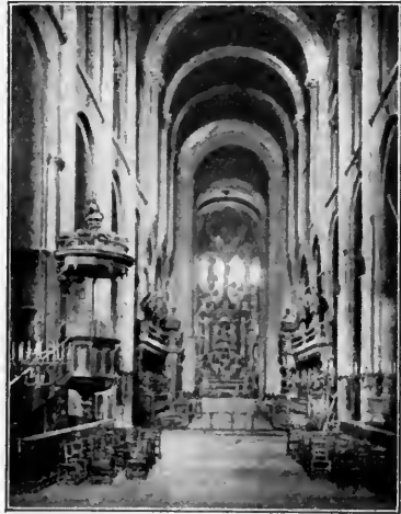
FIG. 122—TOULOUSE. SAINT SERVIN. THE INTERIOR SEEN FROM THE WEST
