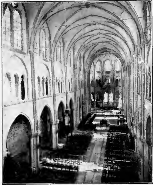
FIG. 146—SAINT LEU D'ESSERENT. VIEW OF THE INTERIOR, SHOWING THE VAULTS AND, THROUGH THE WINDOWS, THE FLYING BUTTRESSES
