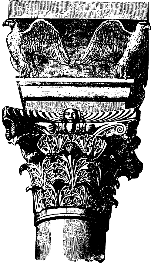
Fig. 153. Column of Marcian, Constantinople.
