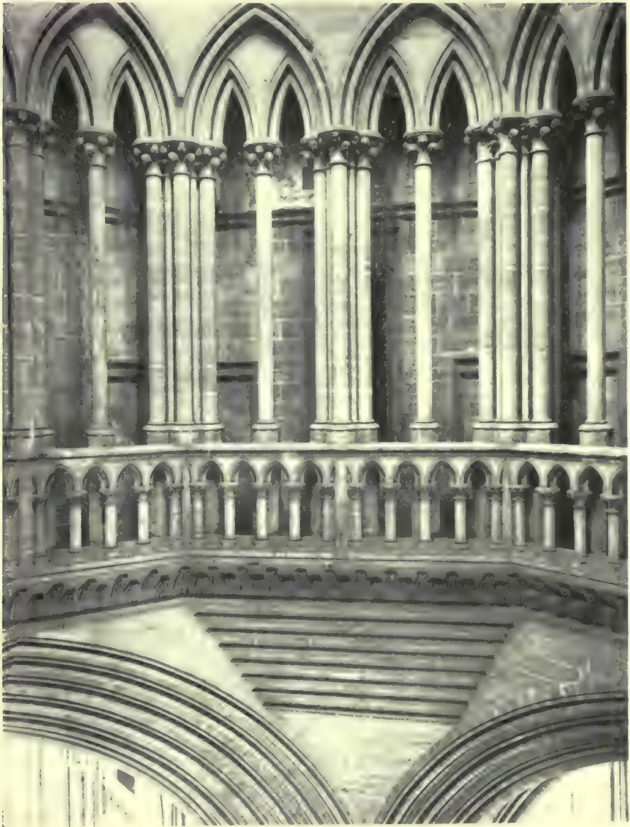
90—Detail of base of lantern, over transept, cathedral of Coutances. (From photo.)
