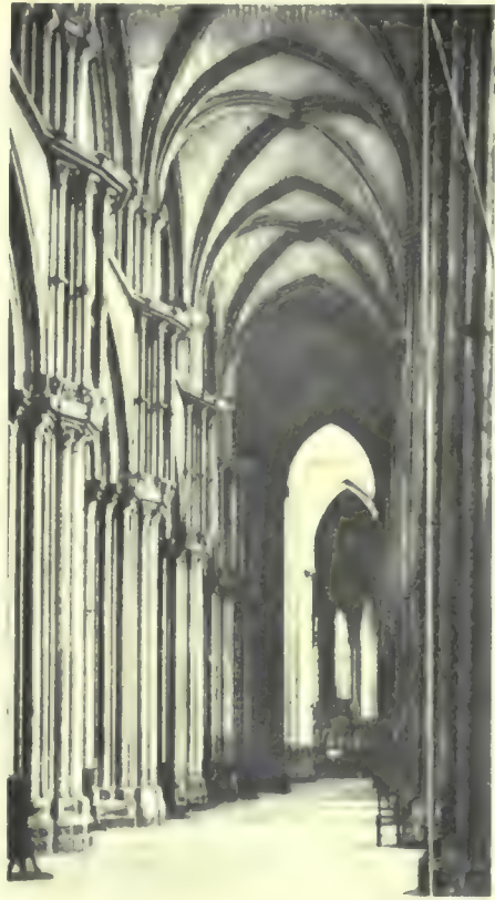
69—Aisle of Rouen cathedral, with plumb line on right, showing widening refinement. (From Mr. Goodyear's photo.)
