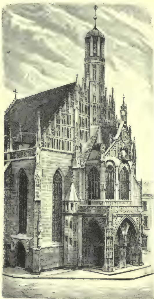
405—Façade of the Frauenkirche, Nuremberg. (From Dohme.)
