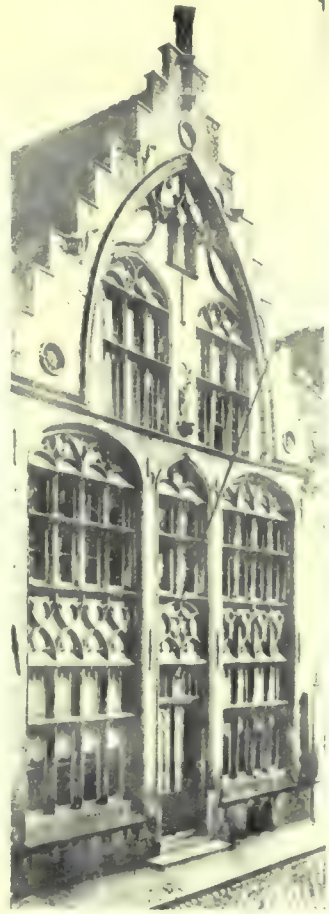
460 House at Bruges. (From Ysendyck.)
