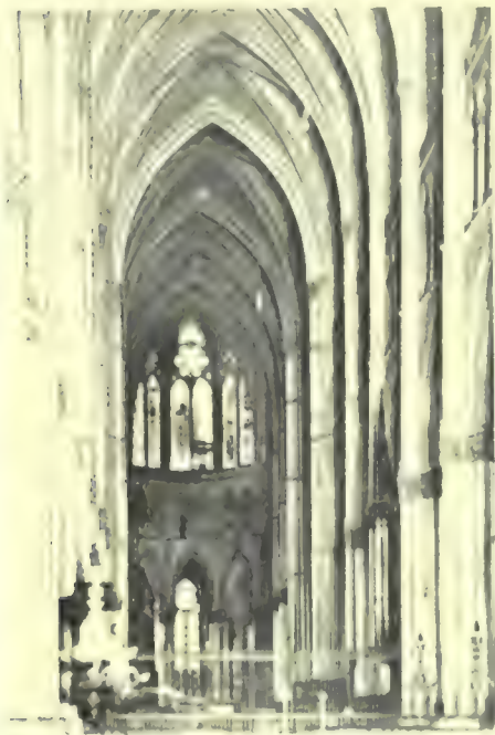
87. Widening refinement of nave of Reims—plumb line on left side. (From Mr. Goodyear's photos.)
