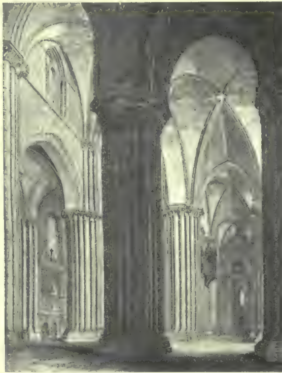
255—Interior of cathedral, Sigüenza. (From Street.)
