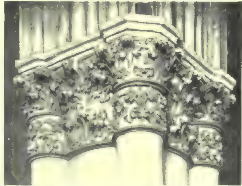
210—Capital of pier of nave, Cathedral of Reims. (From photo.)
