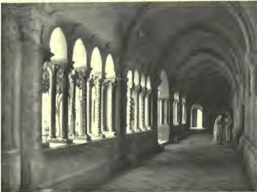
300. Fossanuova monastery, cloister, later section. (From photo.)
