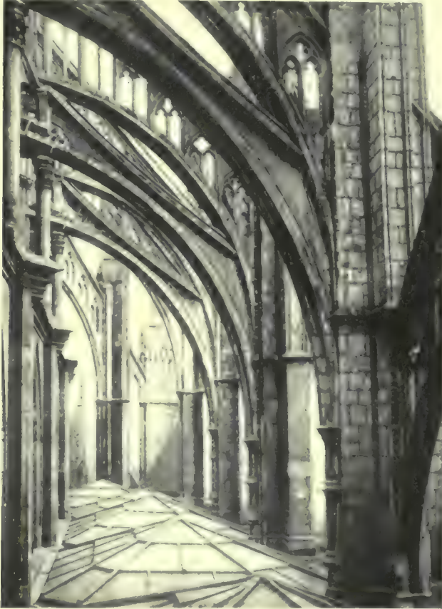
13—Buttress system of nave of Amiens, reinforced with sub-arches, and with open gallery. (From photo.)
