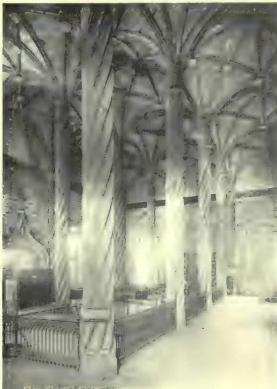
281—Interior of Exchange (Lonja), Valencia. (From Uhde.)
