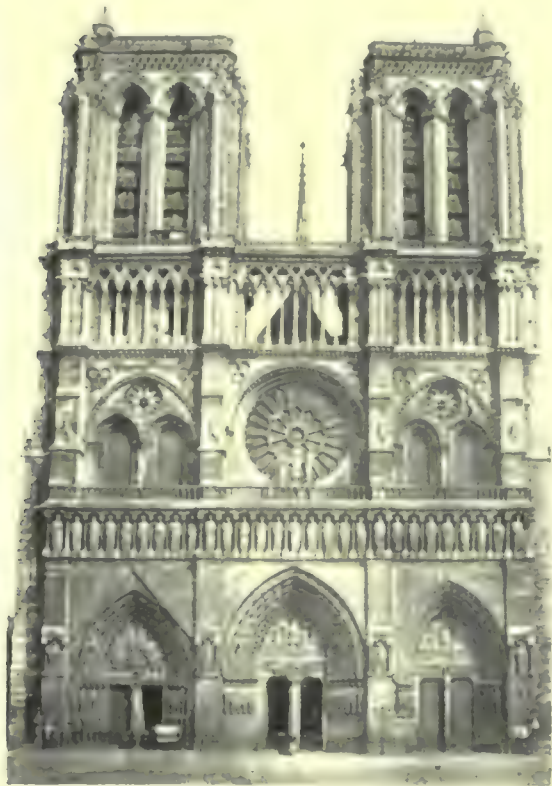
26. West facade of Notre Dame Paris. (From photo.)
