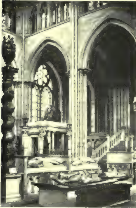
117 —Bays of nave of St. Denis. (From photo.)
