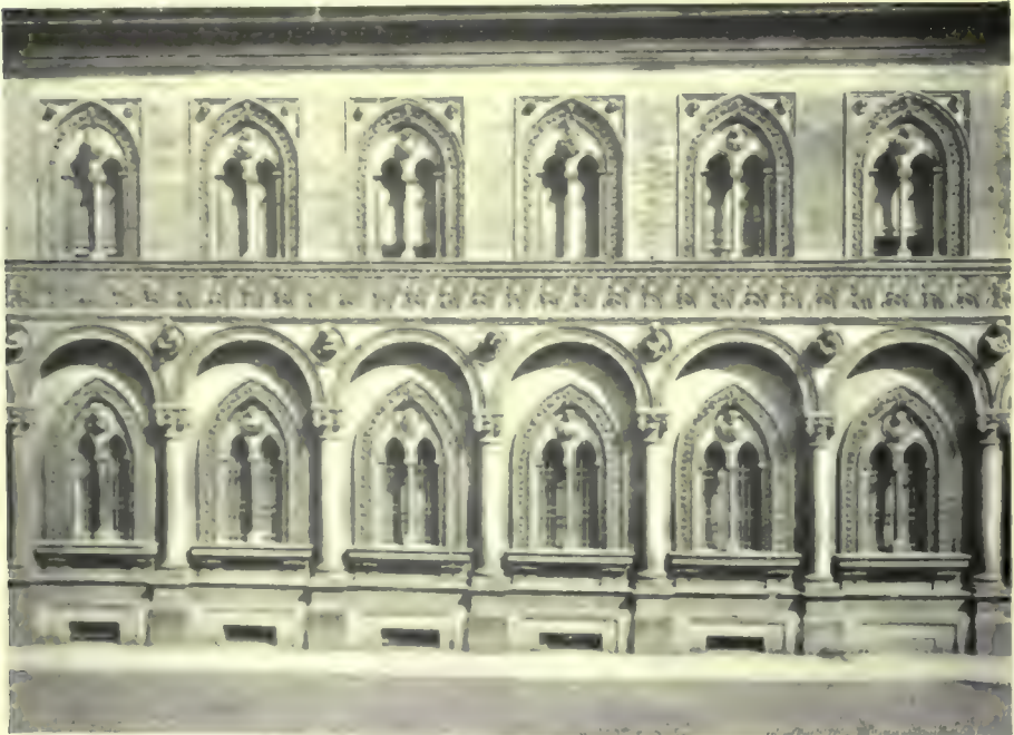
55 Façade of Ospedale Maggiore, Milan. (From Schutz.)
