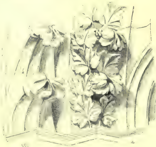
213—Crocket and foliated archivolt in chapter-house of Noyon cathedral. (From Viollet-le-Duc.)
