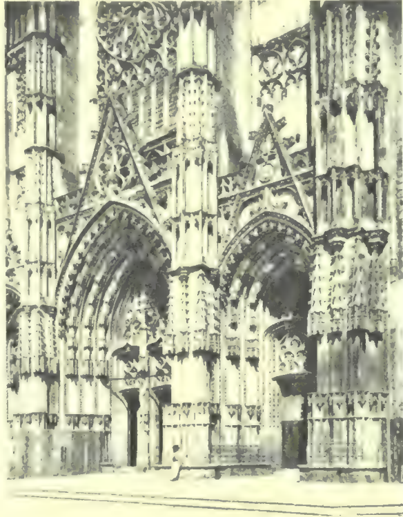
130. West portals of cathedral of Tours. (From Gurlitt.)
