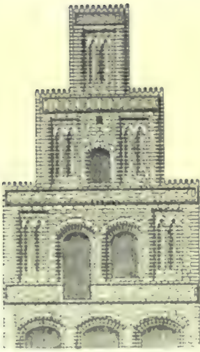
Brick gable end of house at Lateburg. (From Essenwein.)
