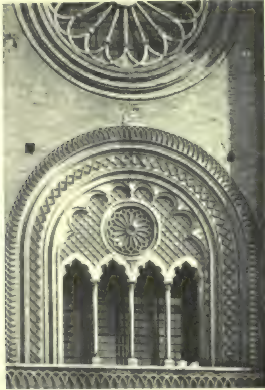
345—Cremona Cathedral: window in minor façade; terracotta detail. (From photo.)
