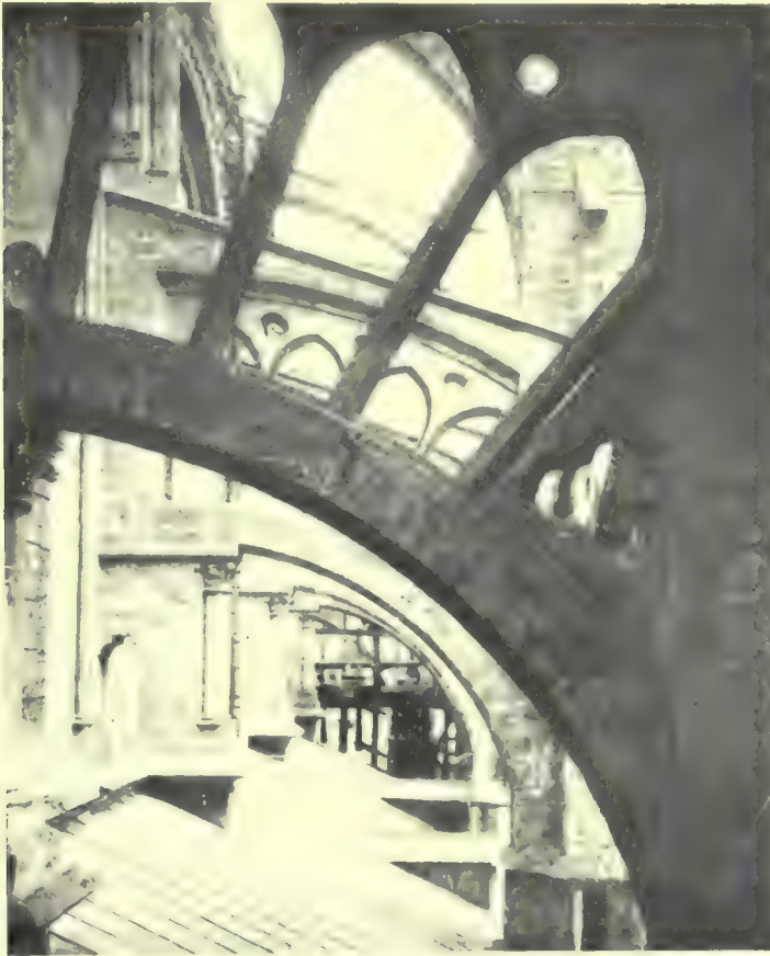
48—Flying buttresses of Chartres cathedral. (From photo.)
