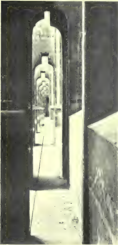
68b—Curve in plan of gallery of Reims cathedral: see surveyor's chain. (From Mr. Goodyear's photo.)
