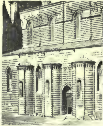
316—Exterior of nave, Orvieto cathedral. (From photo.)
