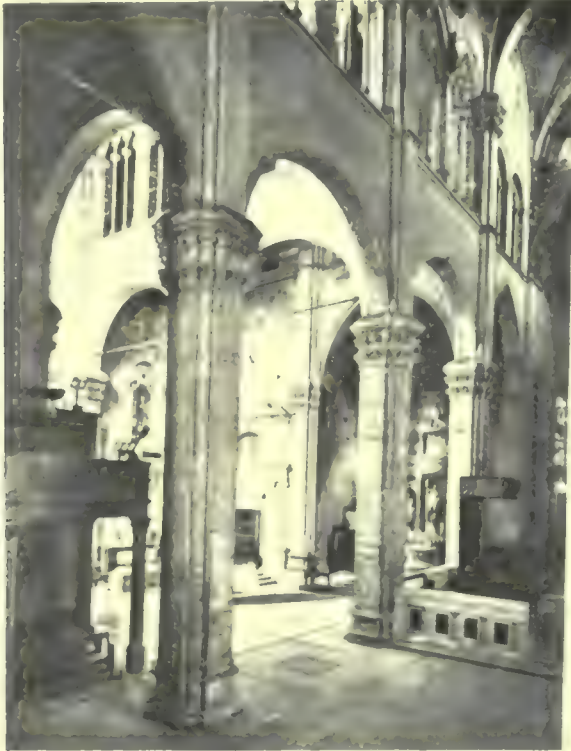
Cathedral of Lucca, view across transept. (From photo.)
