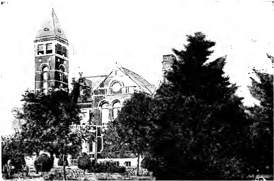
Atchison County High School, Effingham, Kansas
