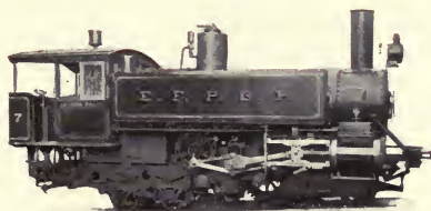
RACK LOCOMOTIVE, WITH TWO COG-WHEELS.
