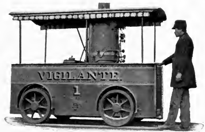
STEAM INSPECTION CAR.
